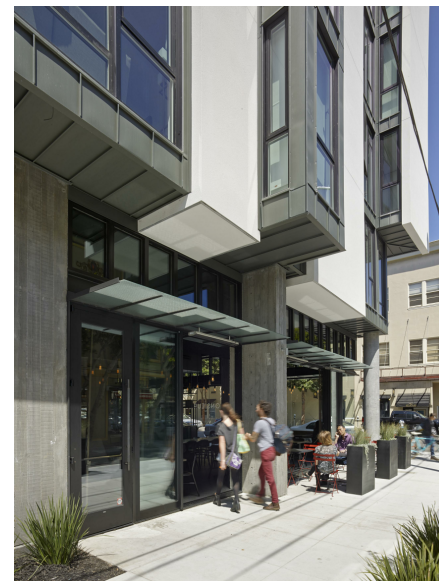
5 STEEL AND GLASS RETAIL AWNING
