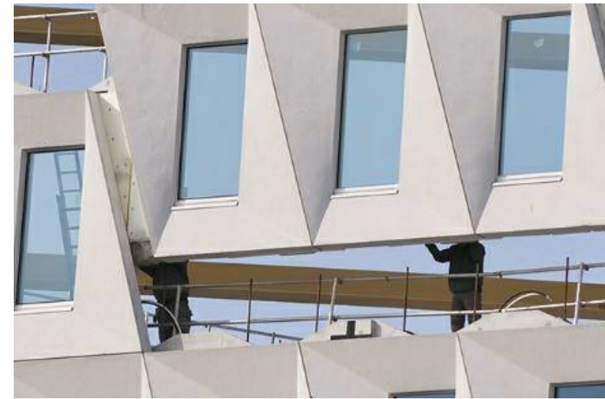
3 GLASS FIBER REINFORCED CONCRETE, 3 COLORS
