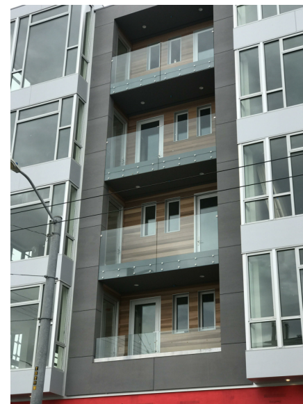
6 GLASS RAILING AT RECESSED BALCONY
