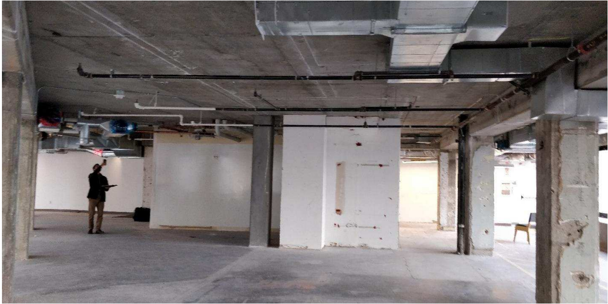
Figure 15 (View of Open Office Space Looking Towards Enclosed Lobby)
