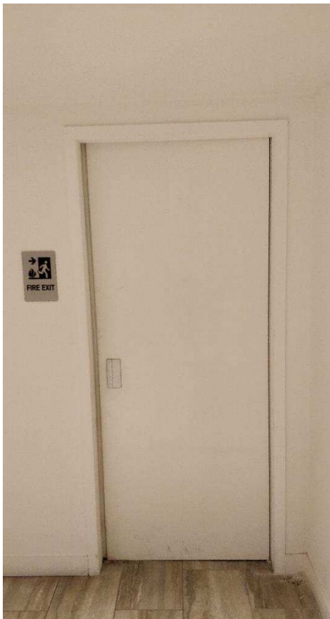
Figure 14 (Door to Tenant Space at 3 rd Floor)
