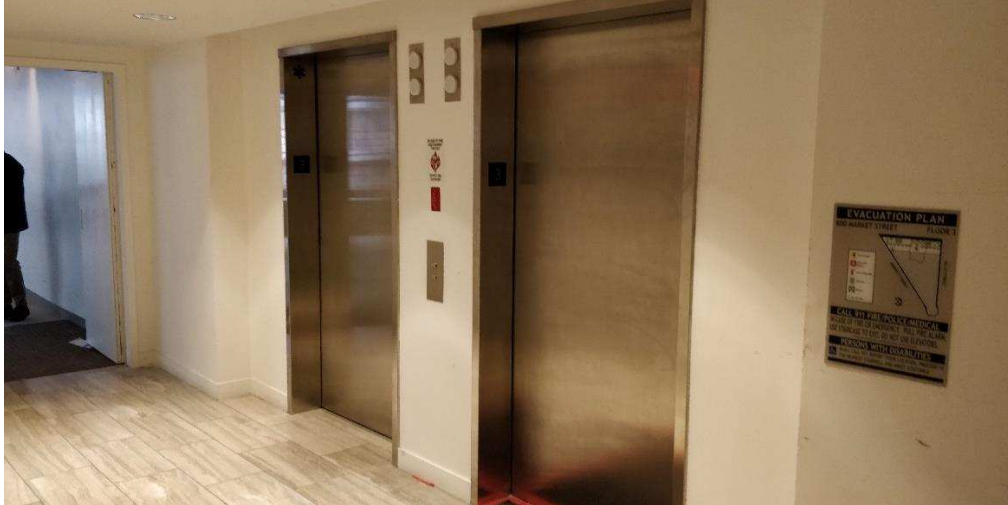
Figure 13 (3 rd Floor Enclosed Elevator Lobby)
