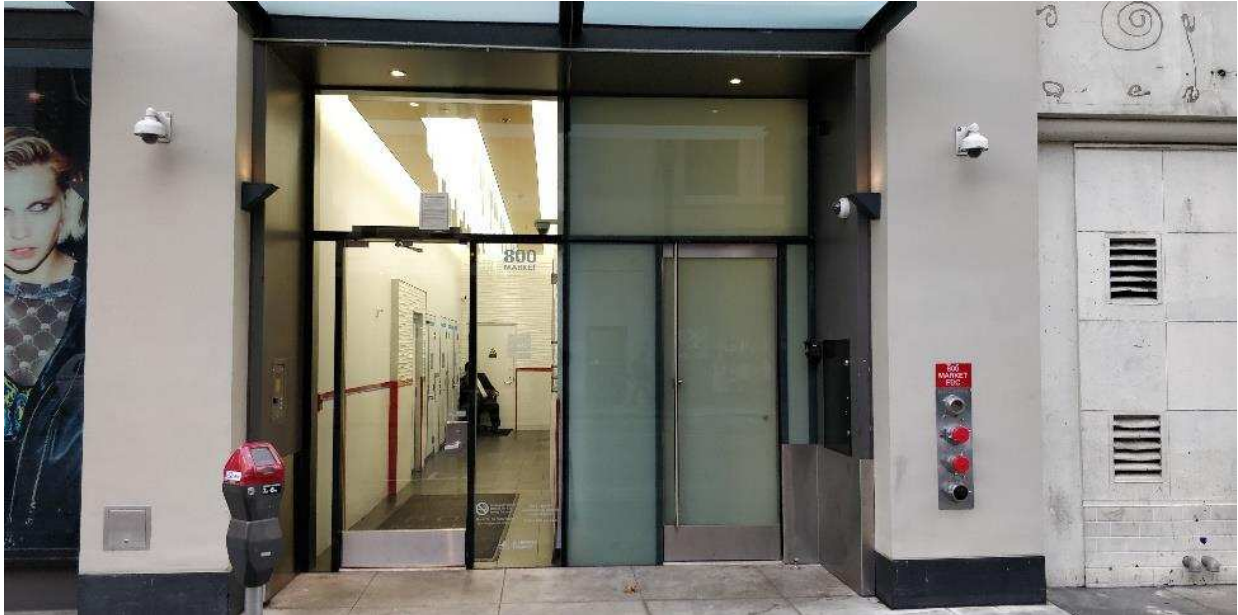
Figure 5 (Main Entry/North Fire Exit Door)
