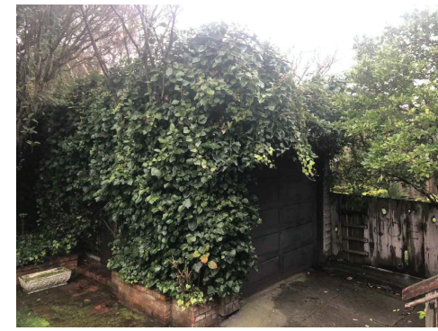
PHOTO 1: EXISTING GARAGE BEFORE DEMOLITION
