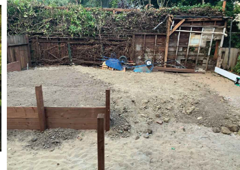
PHOTO 2: EXISTING REAR YARD AFTER DEMOLITION
