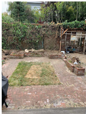
PHOTO 2: EXISTING REAR YARD BEFORE DEMOLITION
