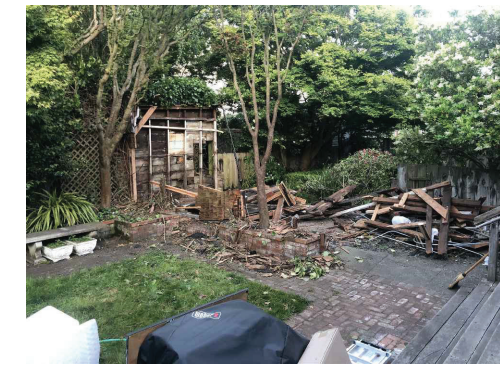
PHOTO 1: EXISTING GARAGE AFTER DEMOLITION
