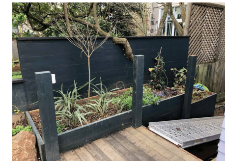
PHOTO 2: AS-BUILT SOUTH & FENCE AND PLANTER BOX
