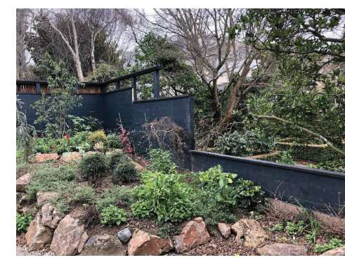
PHOTO 1: AS-BUILT SOUTHEAST CORNER
