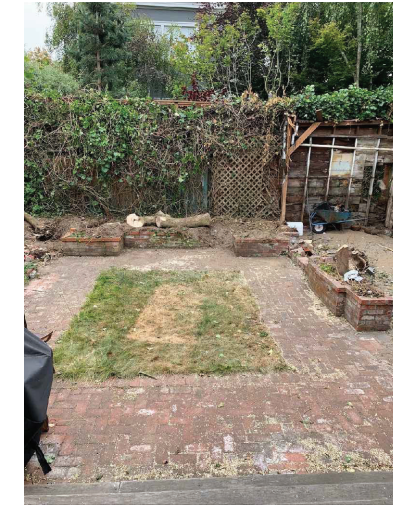
PHOTO 2: EXISTING REAR YARD BEFORE DEMOLITION
