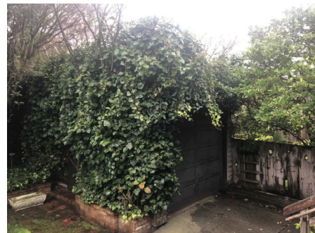
PHOTO 1: EXISTING GARAGE BEFORE DEMOLITION
