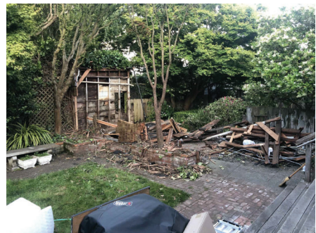
PHOTO 1: EXISTING GARAGE AFTER DEMOLITION
