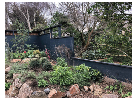
PHOTO 1: AS-BUILT SOUTHEAST CORNER
