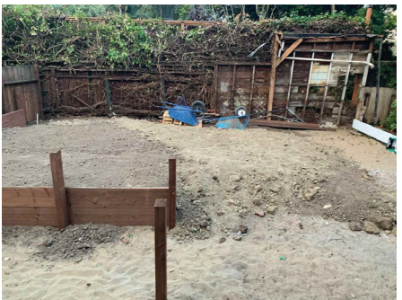
PHOTO 2: EXISTING REAR YARD AFTER DEMOLITION
