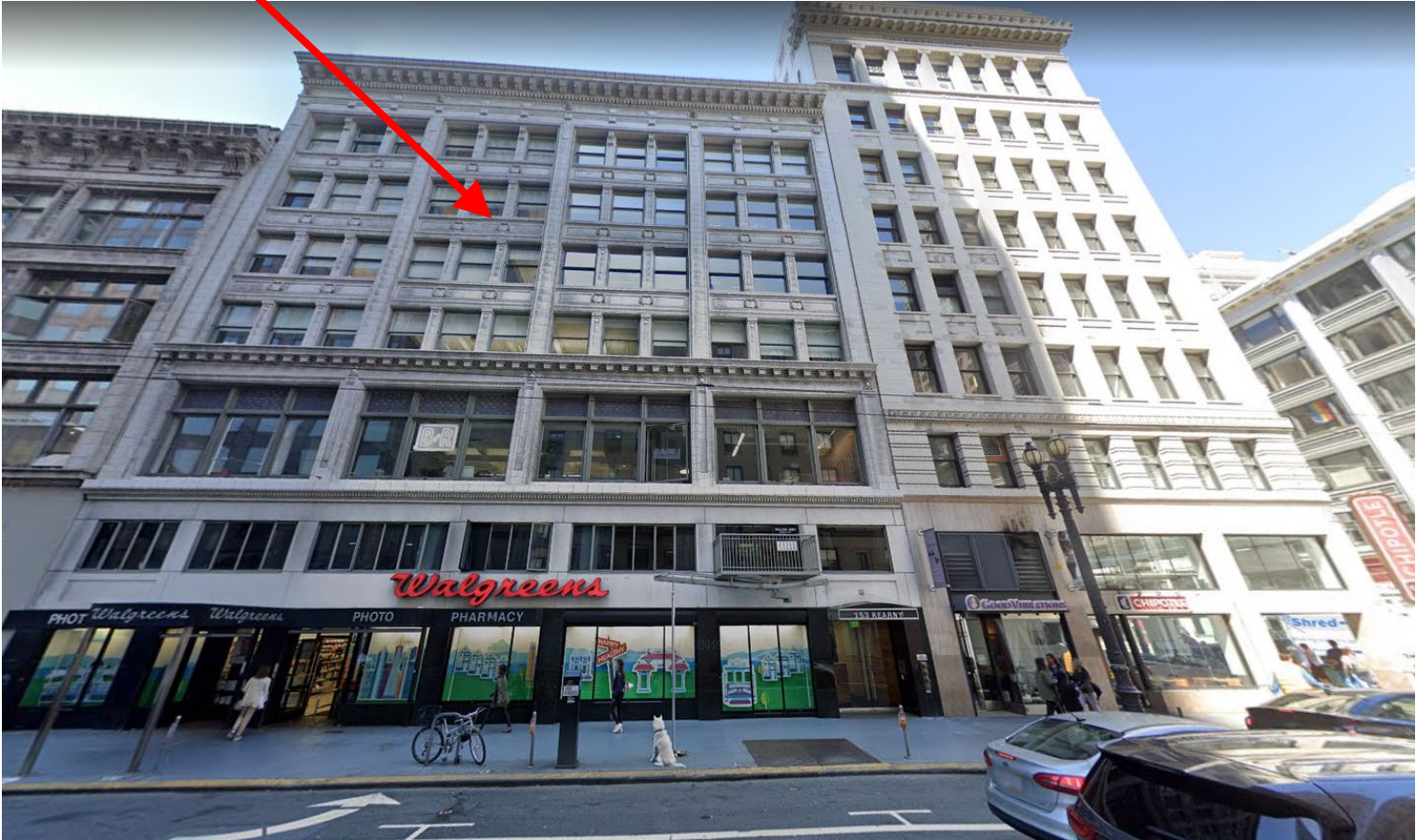
*East (Kearny Street) façade.
