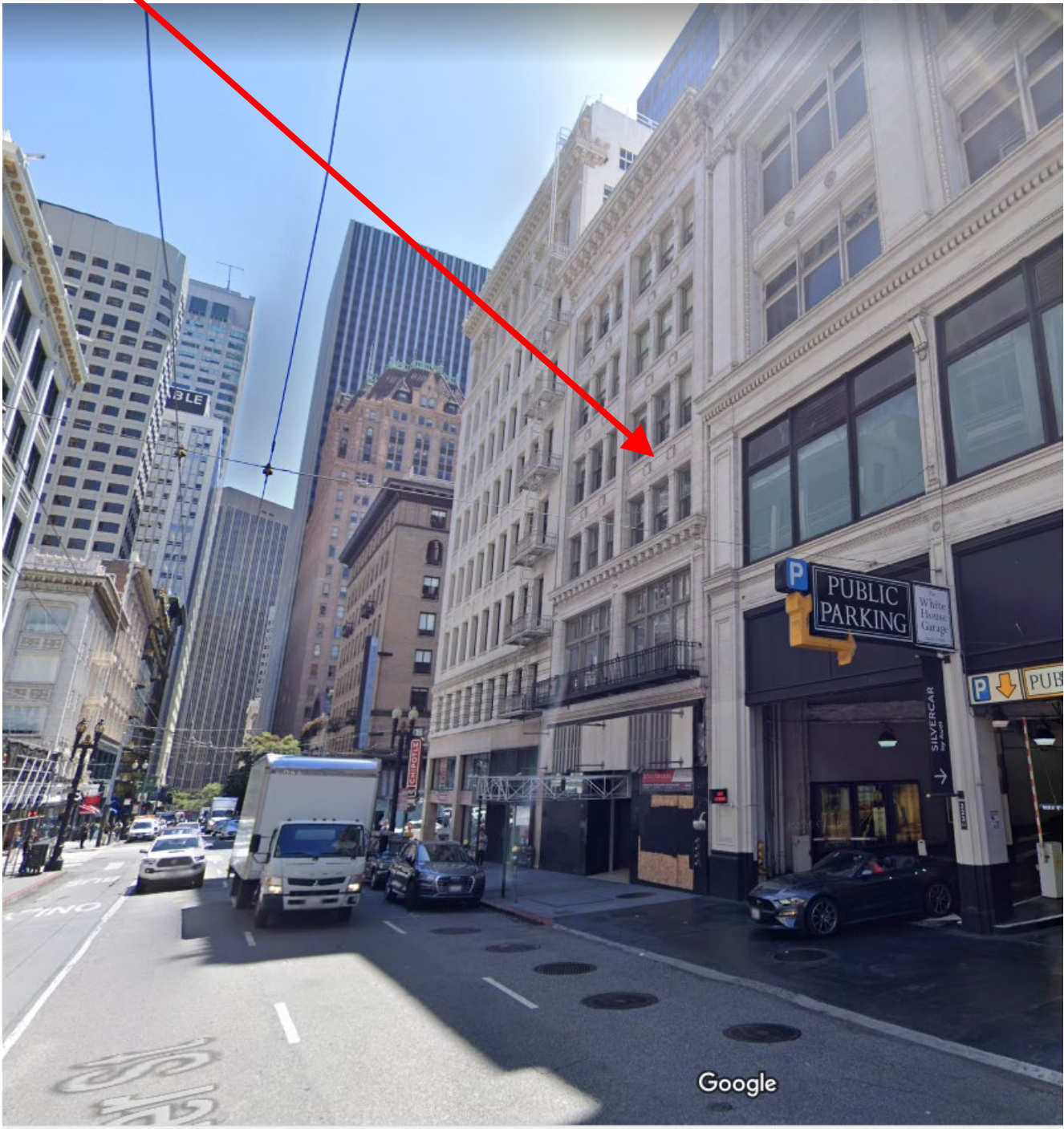
*North (Sutter Street) façade.
