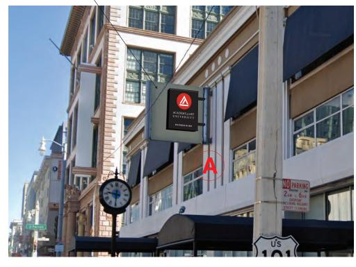
RESIZE PROJECTING SIGN TO CONTAIN CODE-COMPLIANT AAU COPY; RETAIN EXISTING LIGHTING WITH INDIRECT LIGHTING ADDED FOR ILLUMINATION DURING NONBUSINESS HOURS.
