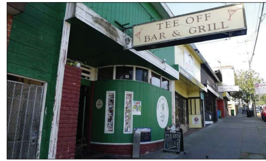
EXISTING EXTERIOR CURVED WALL UNDER WOOD PANELS AT 3129 CLEMENT ST
