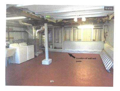
Figure 5. Garage interior – white wall and posts in foreground show the prior eastern extent of the garage which lines up below the rear wall of the house above.
