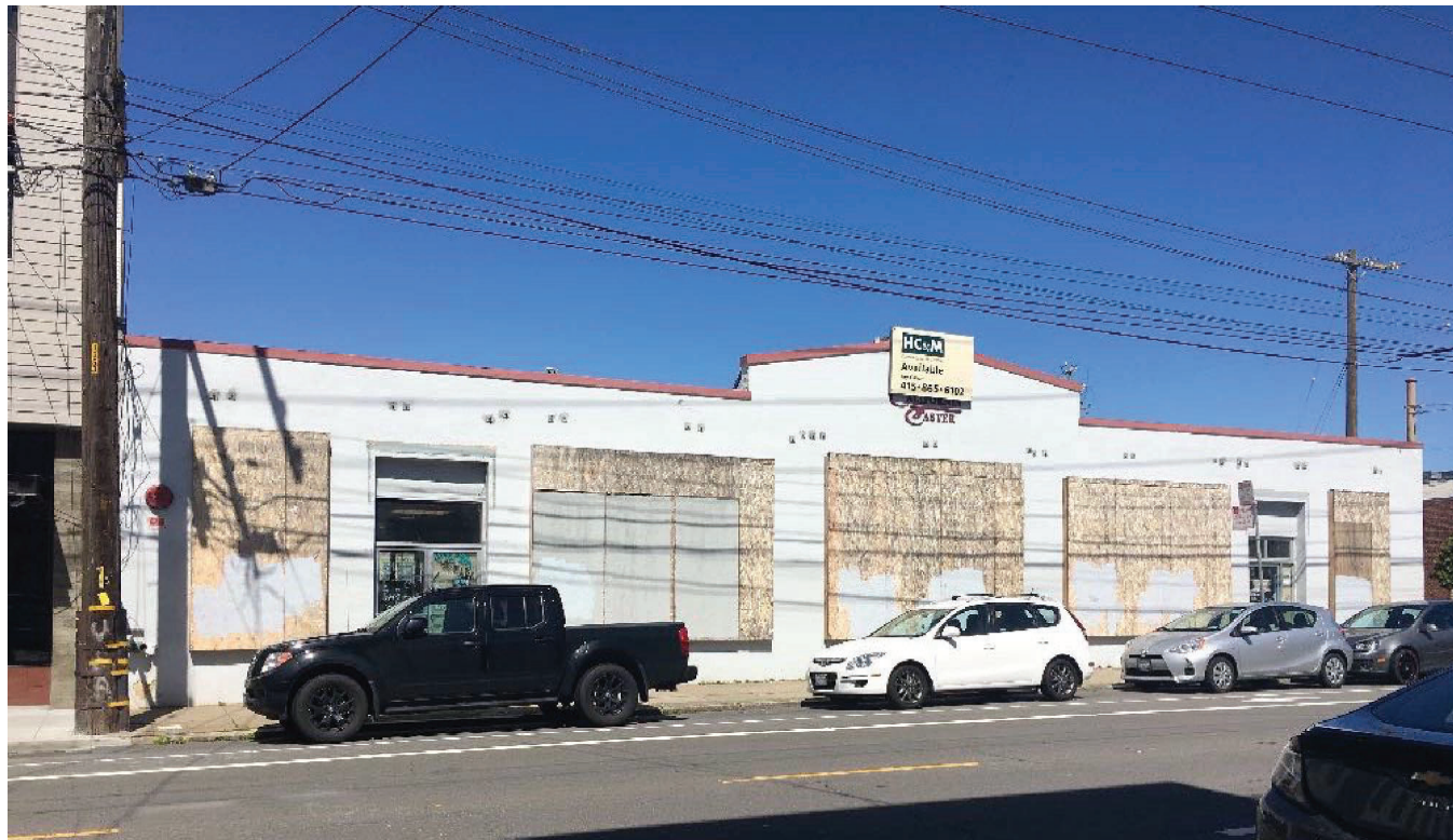
17TH ST (LOOKING NORTH)
