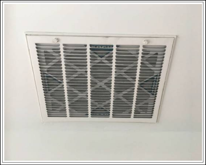
View of Return Air Duct Furnace is in the Attic
