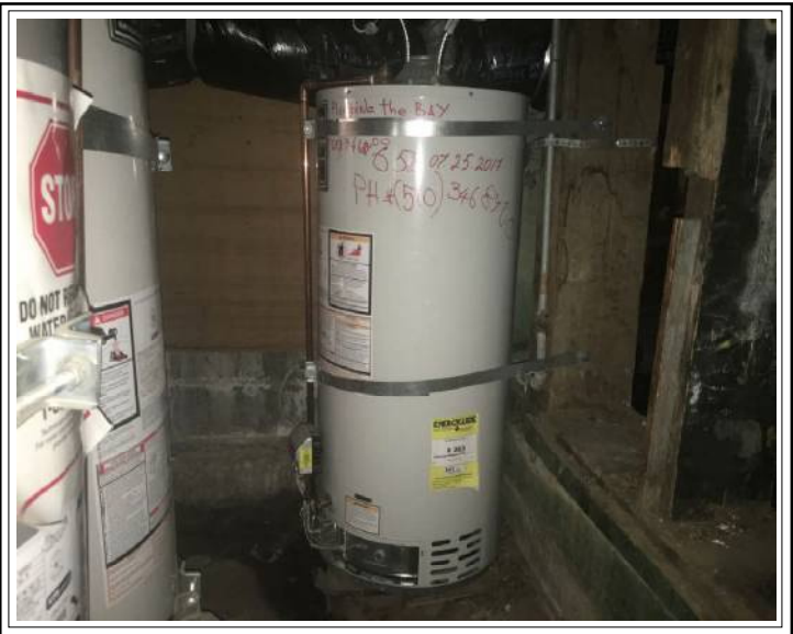
View of the Double Strapped Water Heater
