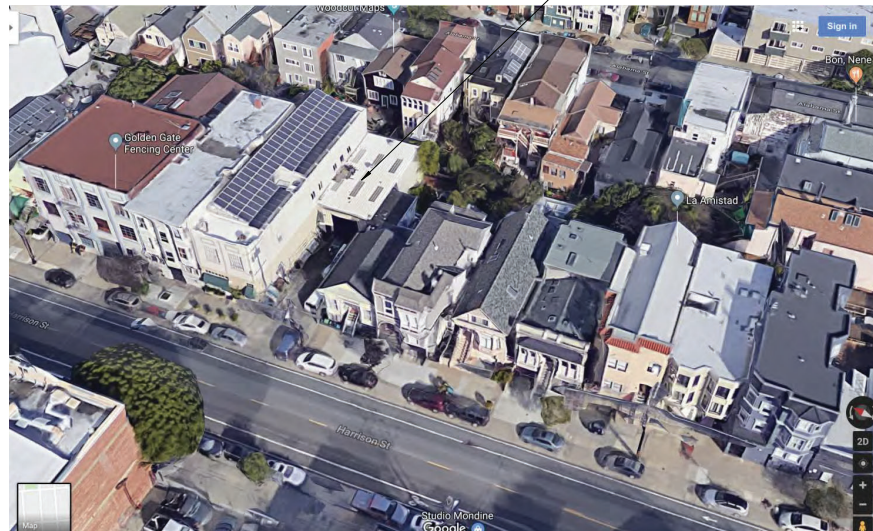
BIRD'S EYE VIEW OF FRONT FACADES
