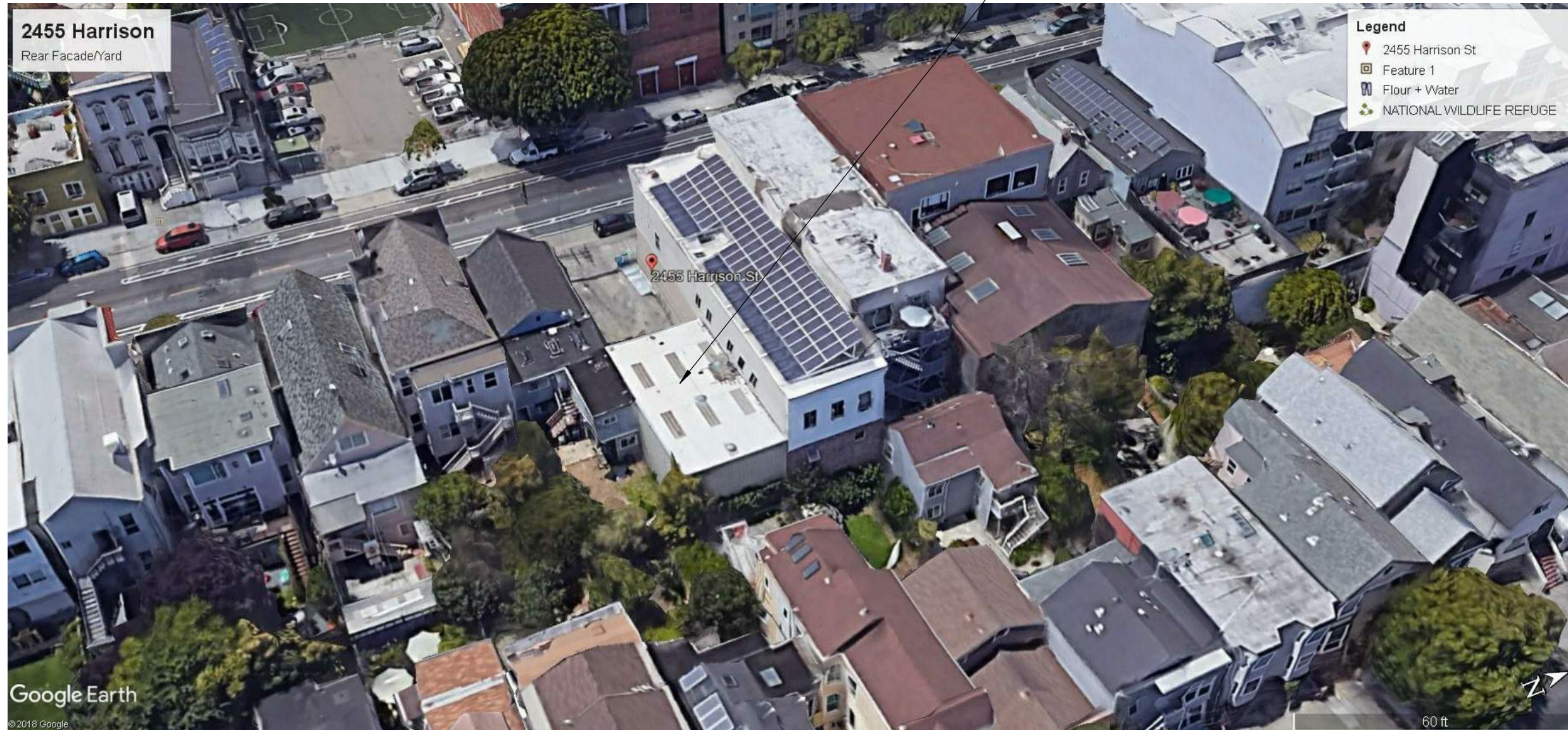
(E) BUILDING AT SUBJECT PROPERTY
