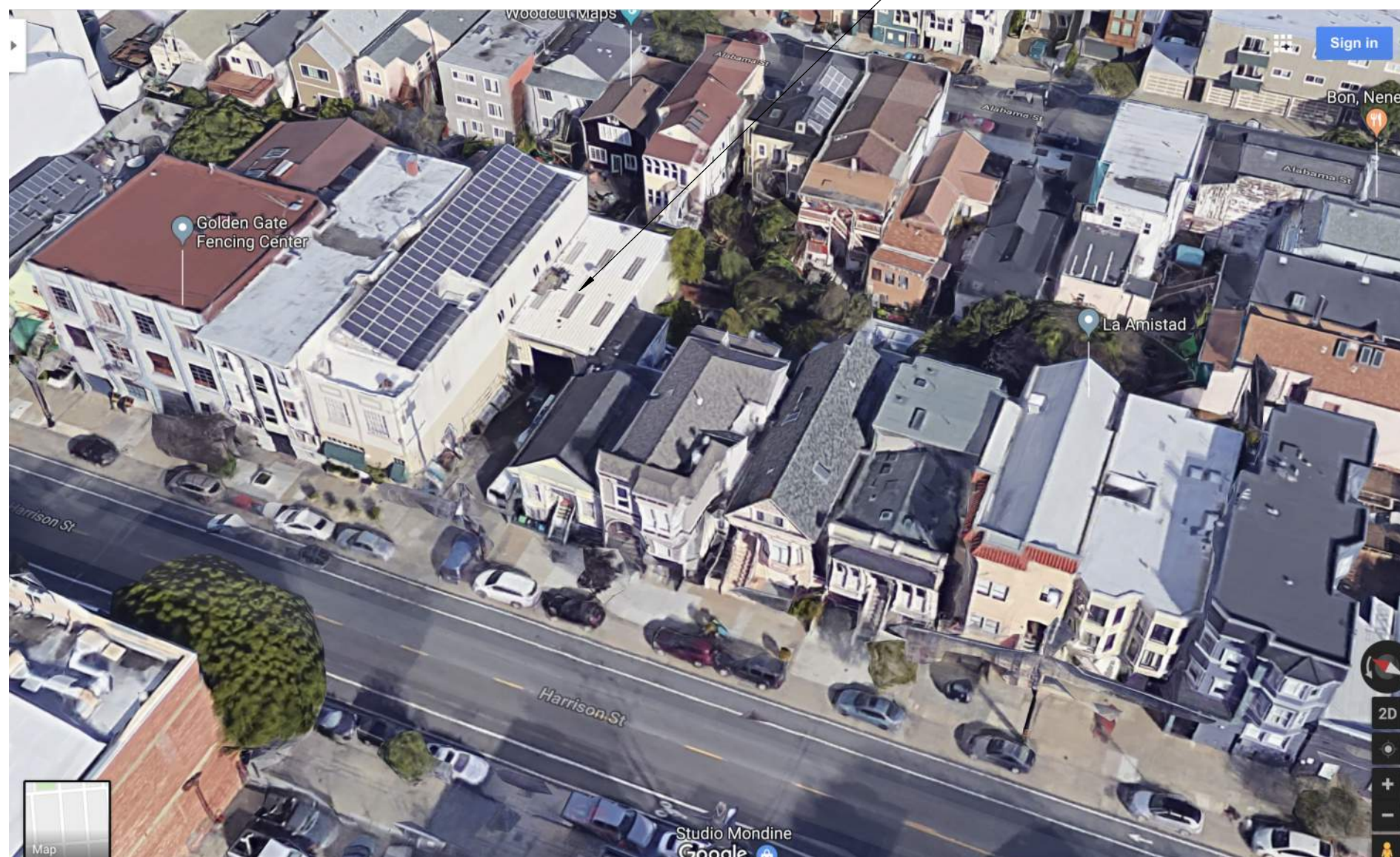
(E) BUILDING AT SUBJECT PROPERTY
