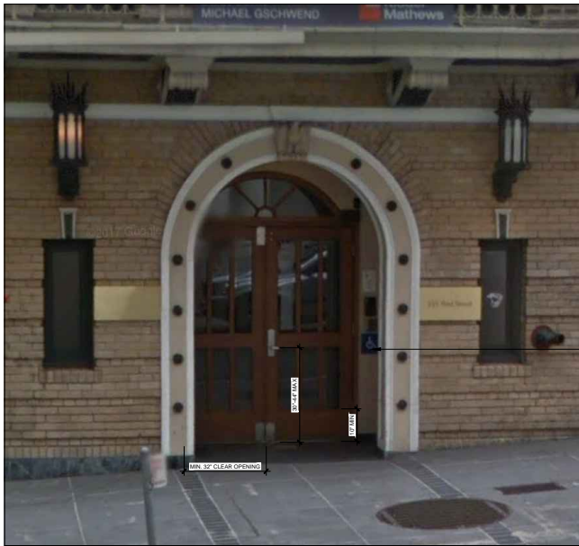
NOTE: EXISTING AUTO OPERATOR TO REMAIN, OPENING FORCE LESS THAN 5 LBS
