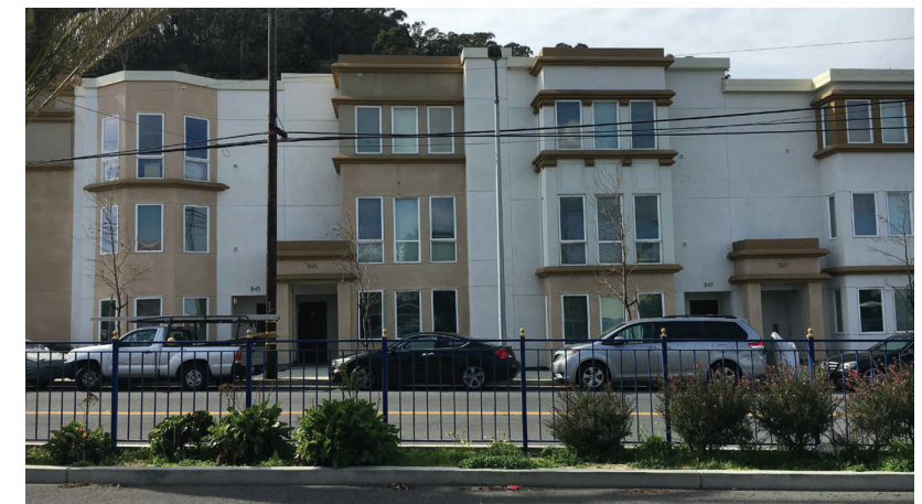
ADJACENT BUILDINGS TO THE NORTH 1
