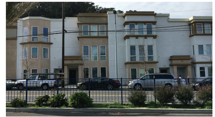
ADJACENT BUILDINGS TO THE NORTH 1
