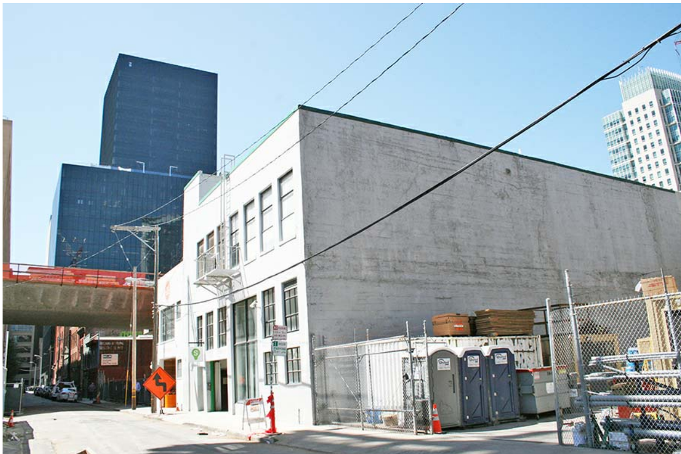
Tehama Looking South
