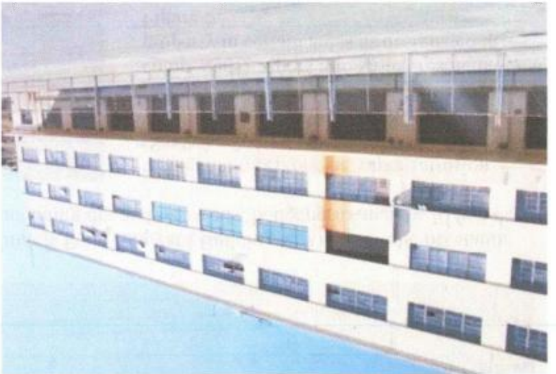
Hunters Point Shipyard Building 813 is a large, 262-by-262-foot, four-story reinforced concrete, flat-roofed building.
