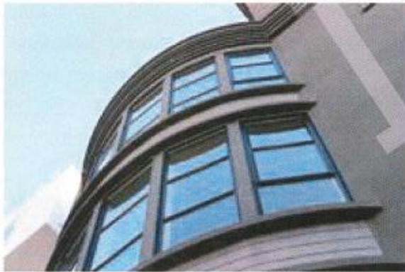
Projecting head and sill trim adds shadow and detail. Vertically proportioned windows with divided lites reflect the prevailing scale of the neighborhood.
