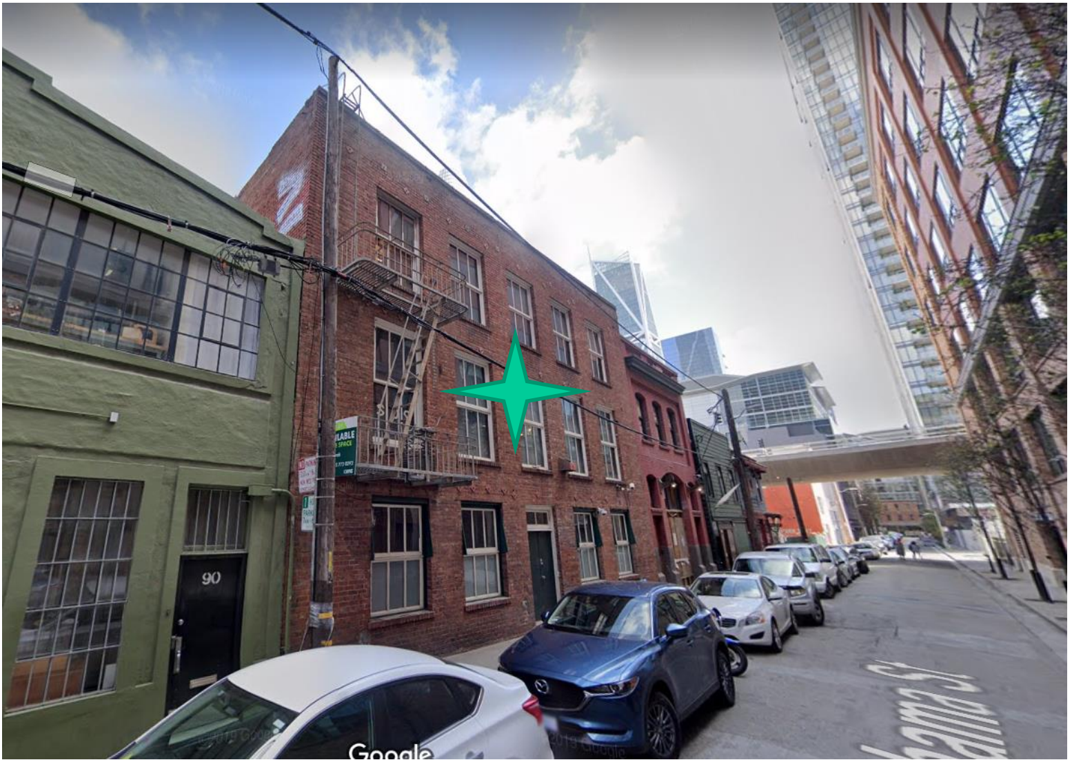
Tehama Street frontage Google Street View – October 2019
