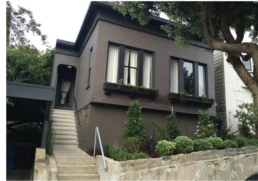
3 SUBJECT PROPERTY - FRONT FACADE
