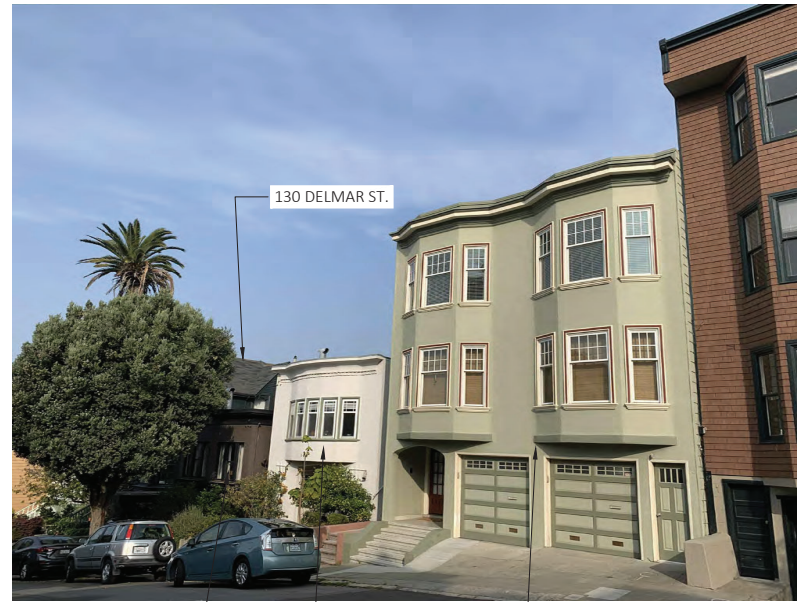
4 STREET ELEVATION - SUBJECT PROPERTY & ADJACENTS
