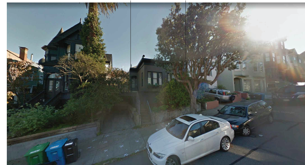
1 STREET ELEVATION - SUBJECT PROPERTY & ADJACENTS
