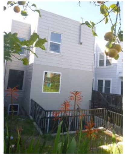
① REAR VIEW TO NORTH
