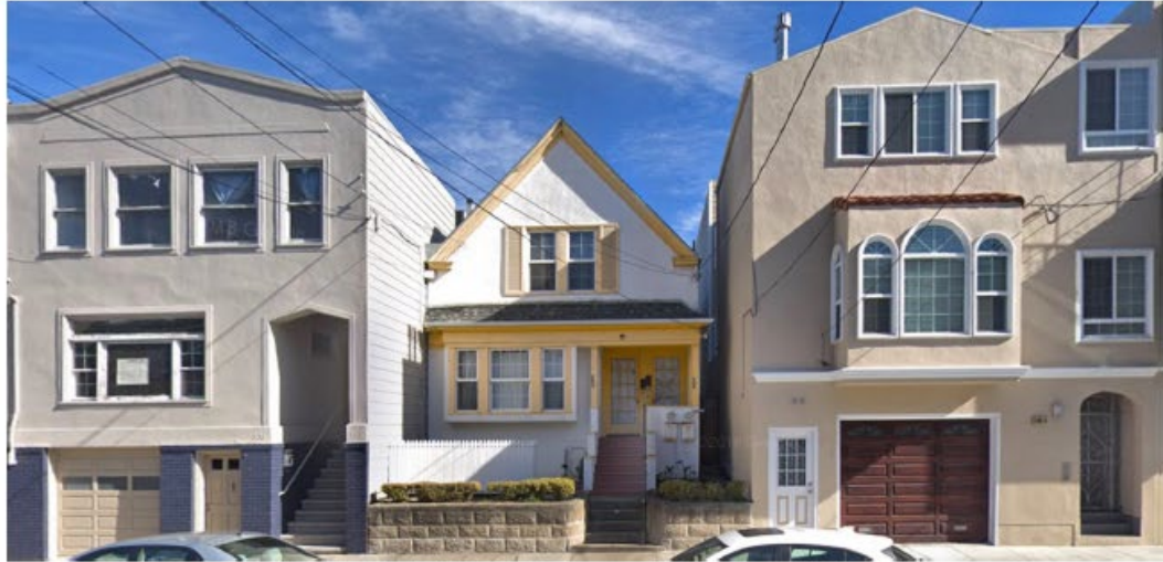
④ EXISTING FRONT VIEW
