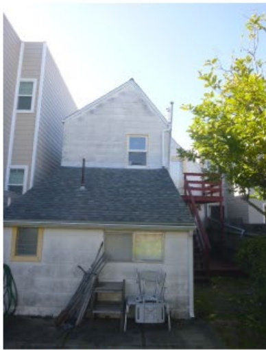
② EXISTING REAR VIEW
