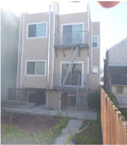
③ REAR VIEW TO SOUTH
