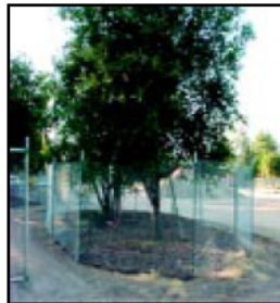
IMAGE 2.15-1 Tree Protection Fence at the Dripline
