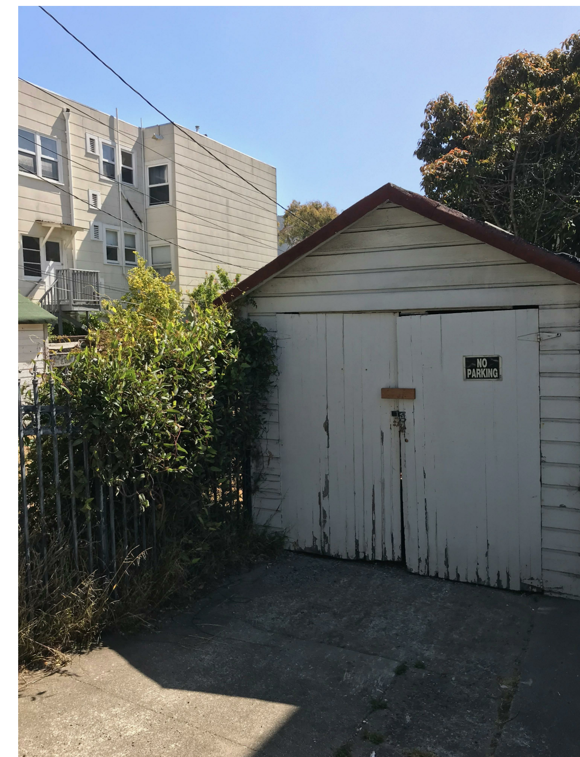
EXISTING GARAGE AT 1222 FUNSTON TO DEMOLISH
