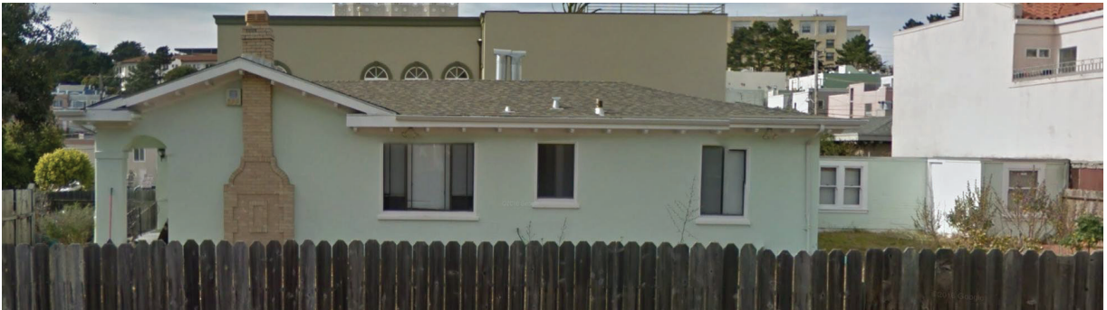
Figure 2 - 492 45th Avenue, South Facade. Google Maps, 2017
