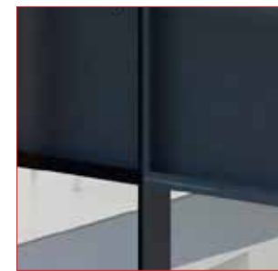
2 Shadow Box: Glass Coating to Match Upper Level North Glazing Solarban 60 Custom Paint for Shadow Box
