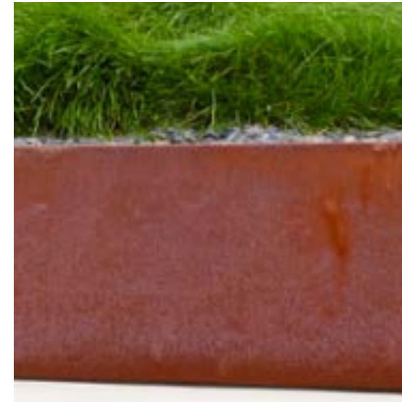
Weathered Steel edging
