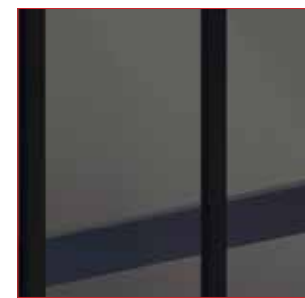
1 Upper Level Glazing (North Excluded): Halio Glass
