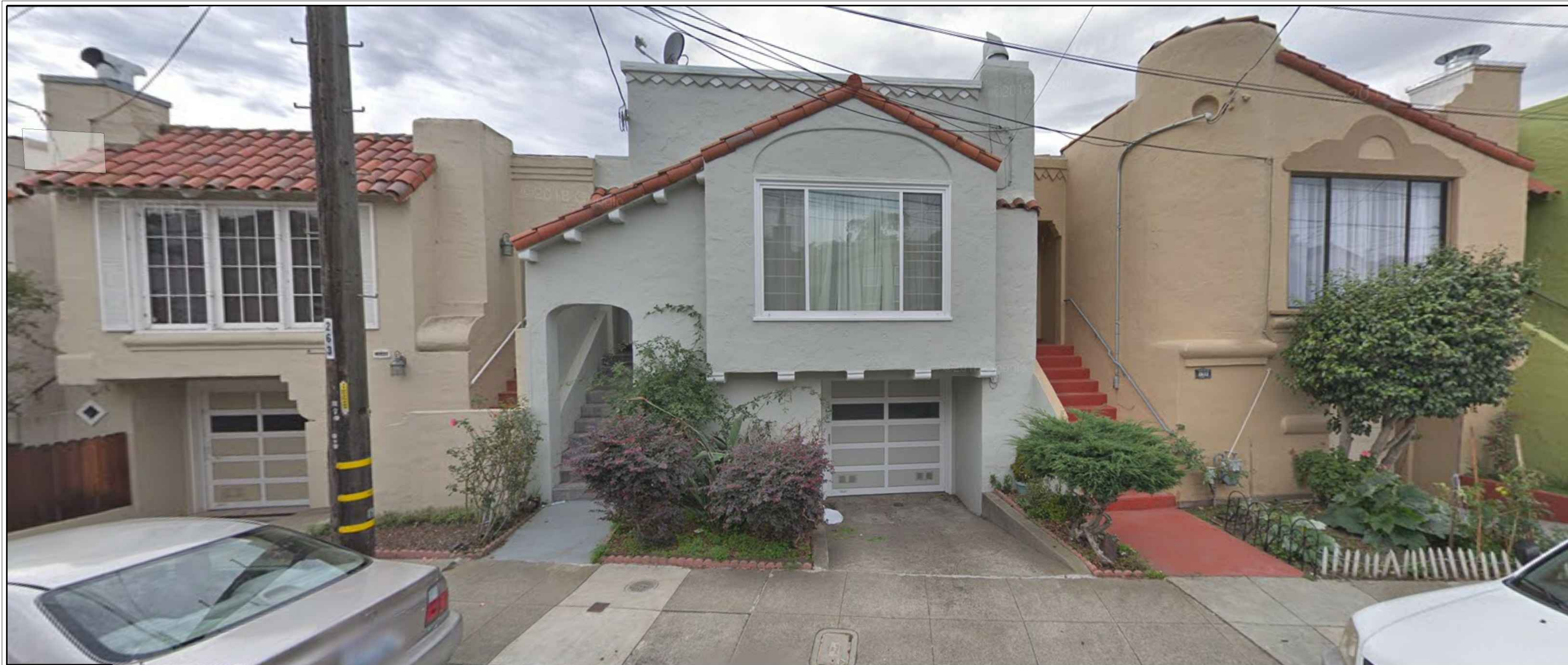
3 FRONT ELEVATION PHOTOS
