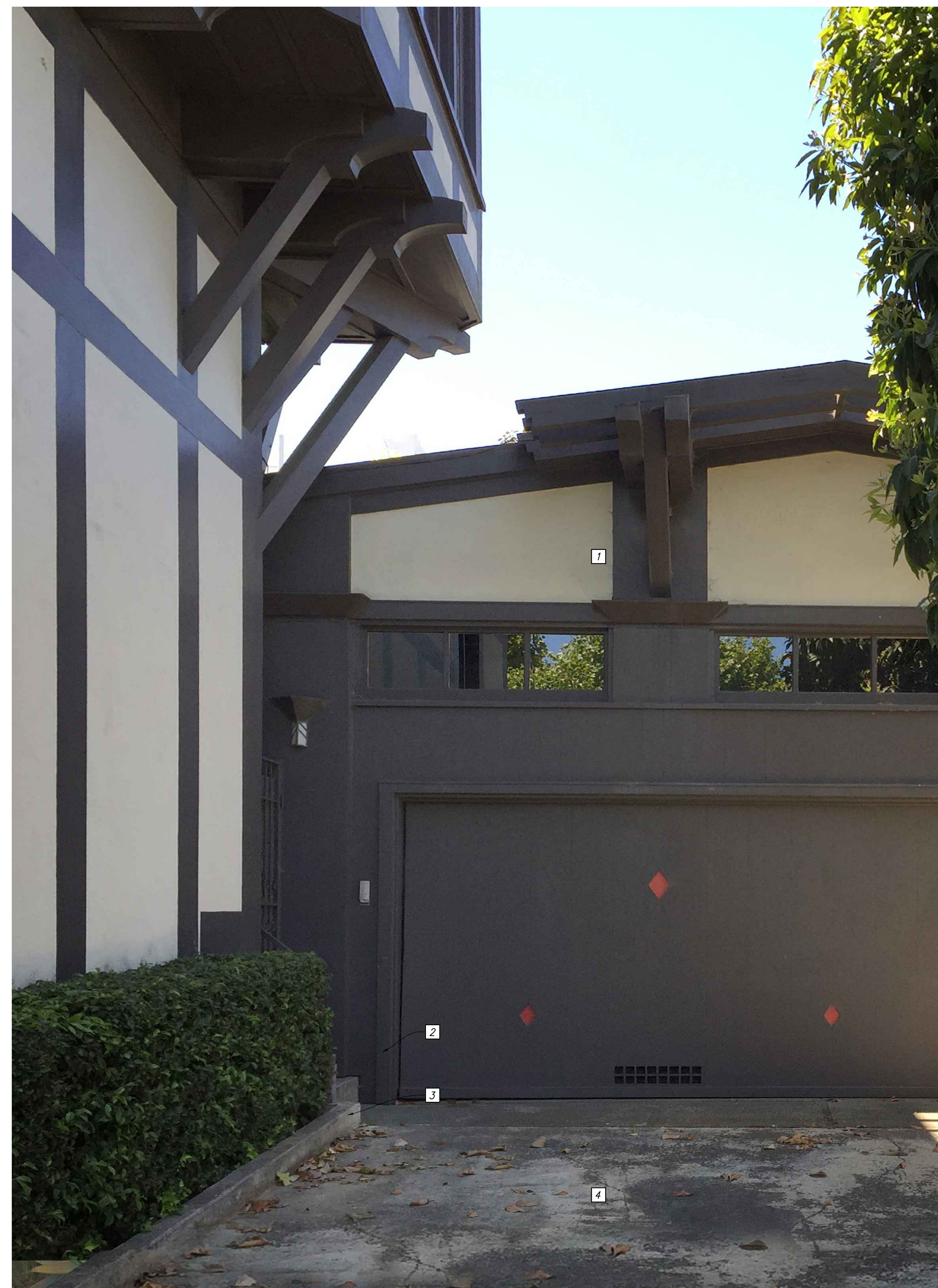
2 PHOTO: EXISTING GARAGE SCALE: NTS
