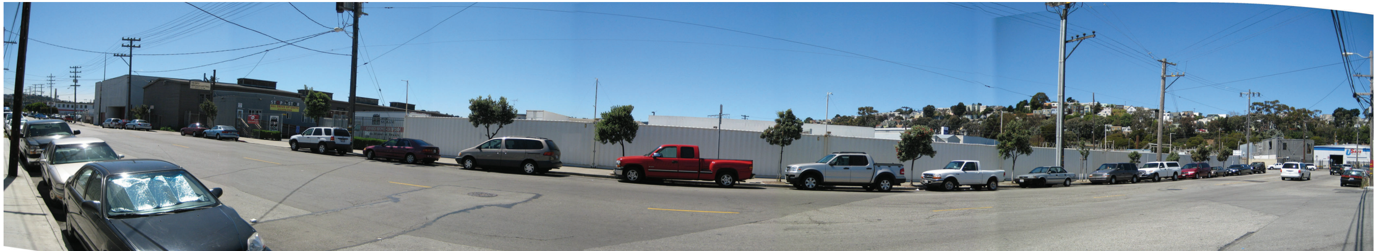
VIEW FROM ACROSS JERROLD TOWARD SITE
