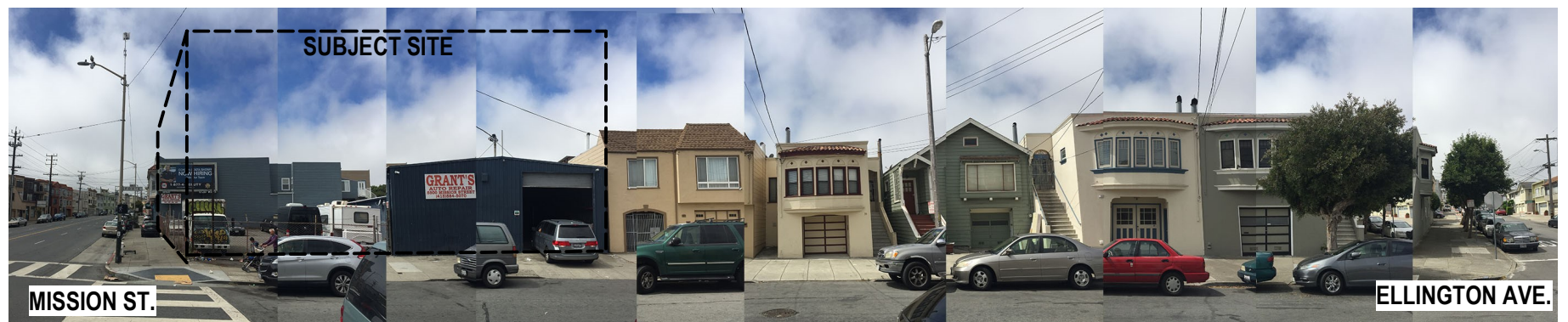
SUBJECT AND ADJACENT BUILDINGS ON FOOTE AVENUE
