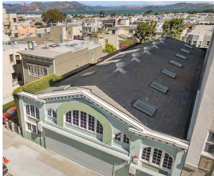
2 FRONT BUILDING FACADE & ROOF
