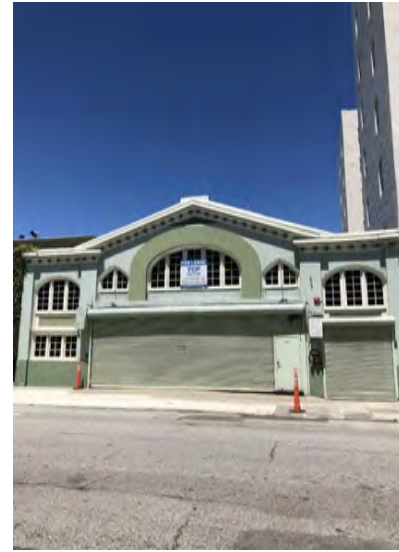
3 1776 GREEN ST. SUBJECT PROPERTY
