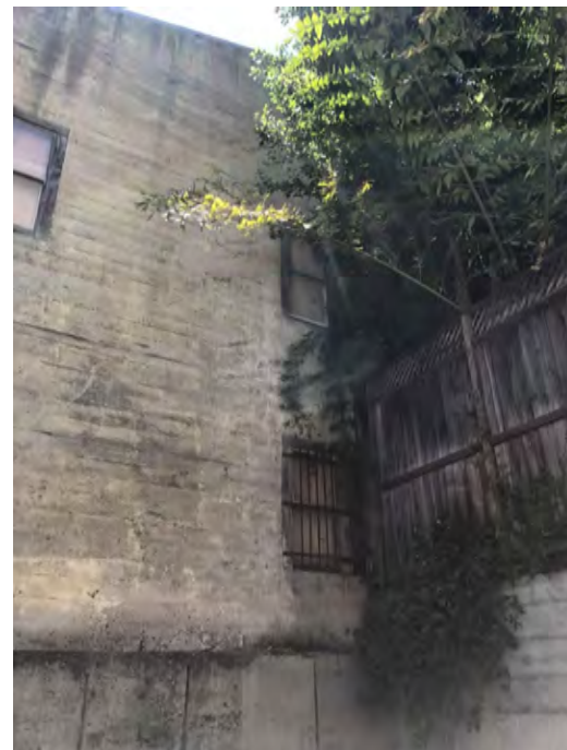
5 REAR FACADE BLOCKED BY ADJ. BLDG.
