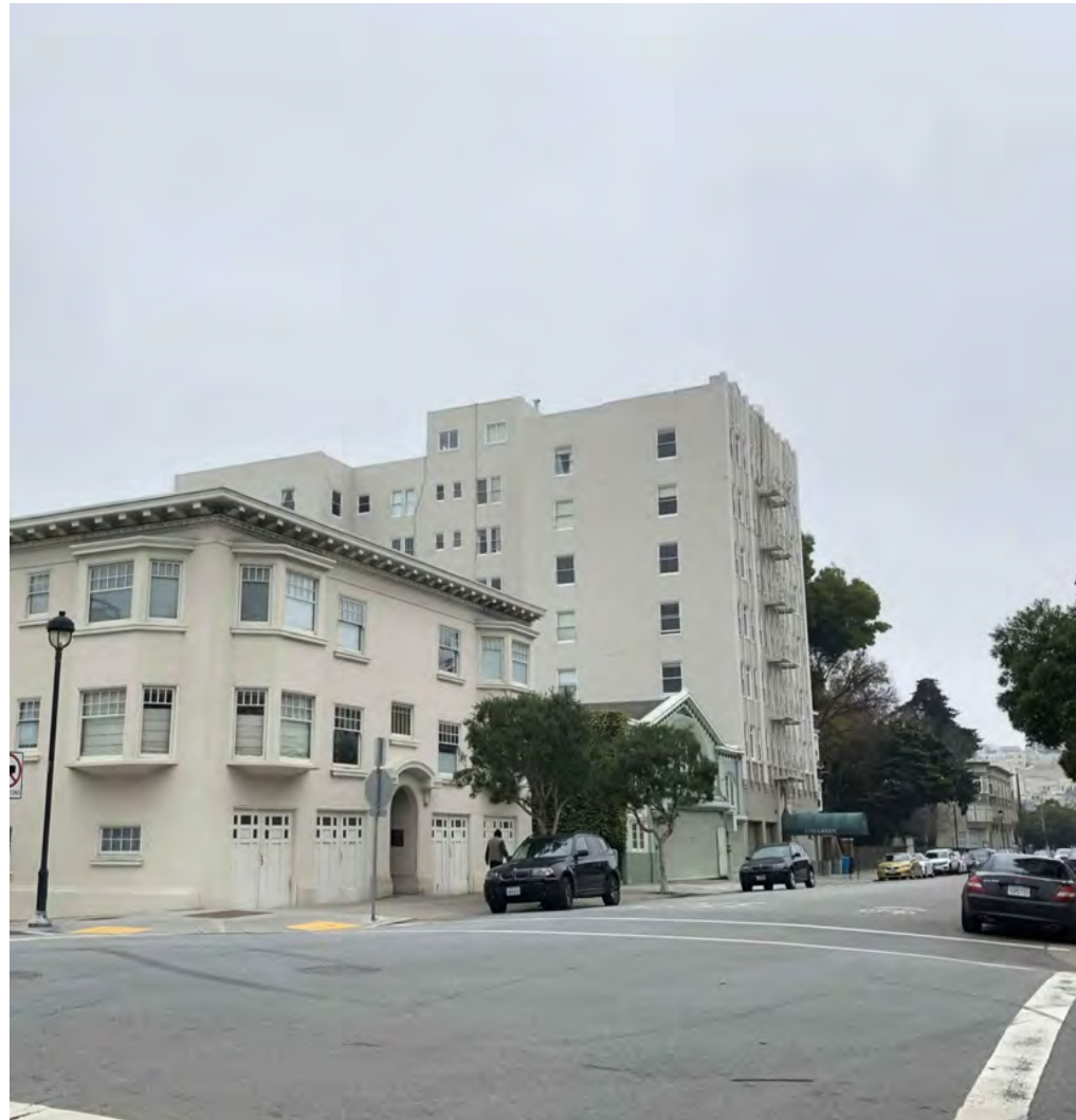
2 EXISTING VIEW 02 - VIEW FROM +/- 150 FEET SOUTHWEST OF SUBJECT PROPERTY
