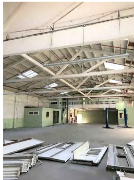
6 INTERIOR OF BUILDING AT FIRST FLOOR
