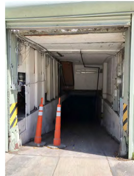
3 PARKING ENTRANCE AT FRONT FACADE
