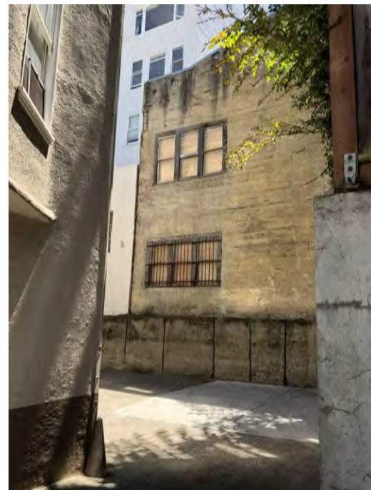
4 REAR BUILDING FACADE
