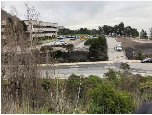
VIEW OF EXECUTIVE PARKWAY FROM POLE LOCATION
