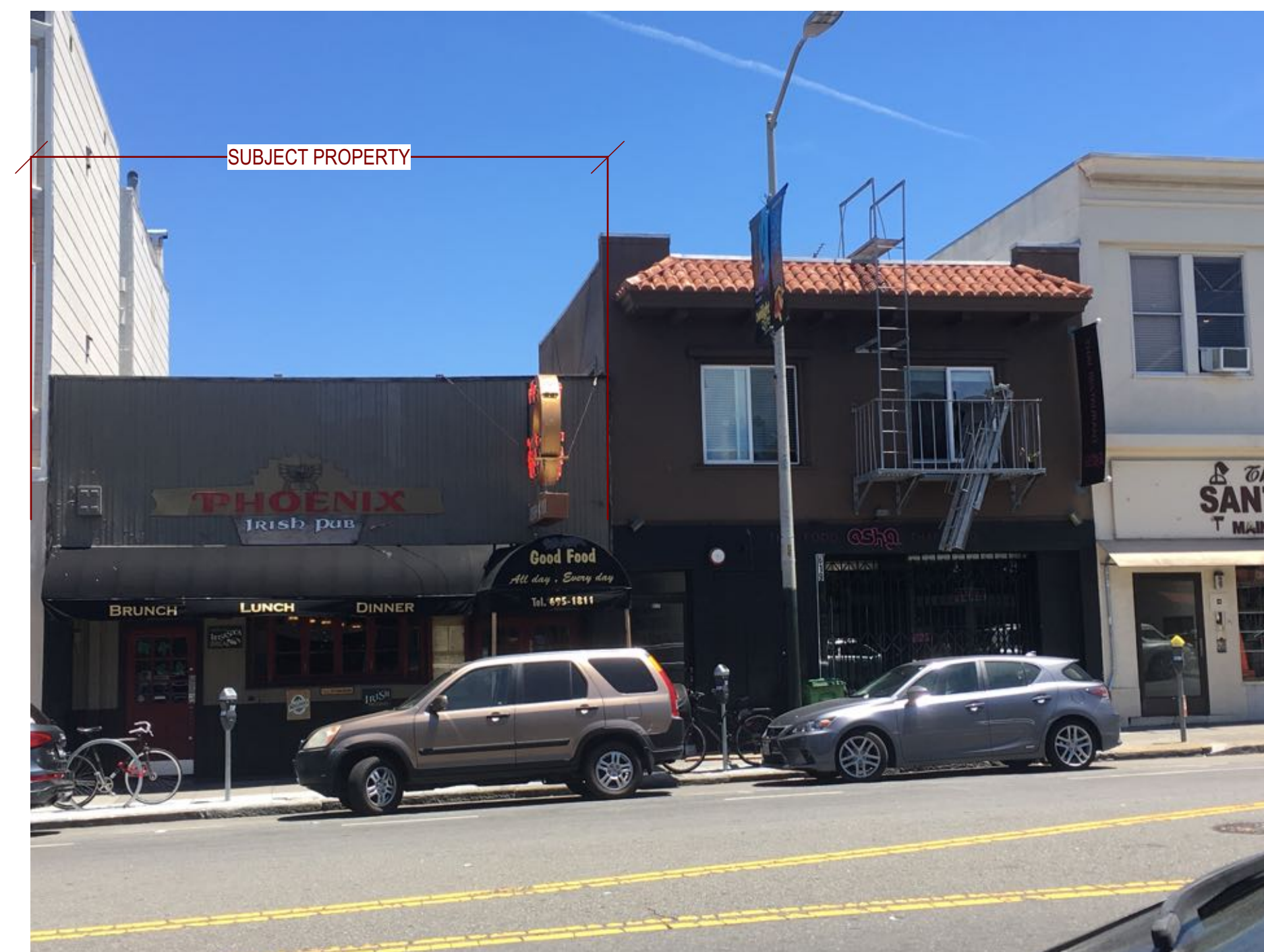
PROPERTY TO THE RIGHT OF SUBJECT PROPERTY
