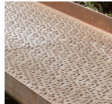
Slip-resistant weathered steel decking at rain garden elevated walkway
