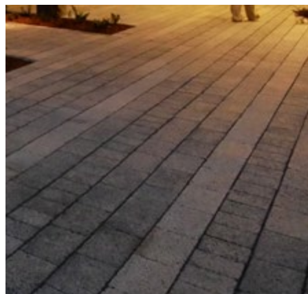
Pervious concrete unit pavers at plaza
