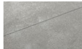
CIP Concrete ; Natural Gray w/ Silica Carbide & Water Jet Finish
