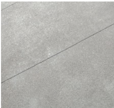
Cast-in-place concrete with silicon carbide and saw-cut joints at pathway
