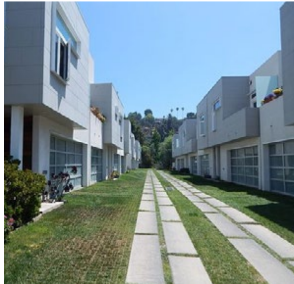
Figure 5.16-2: Permeable and vehicular rated paving is used to maximize pervious surface for stormwater management
