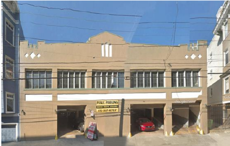
(The existing public parking garage at the Property)
