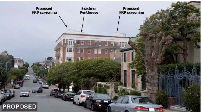
Install (16) panel antennas inside proposed FRP screening on existing rooftop
