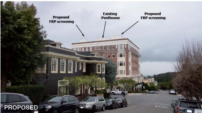
Install (16) panel antennas inside proposed FRP screening on existing rooftop
