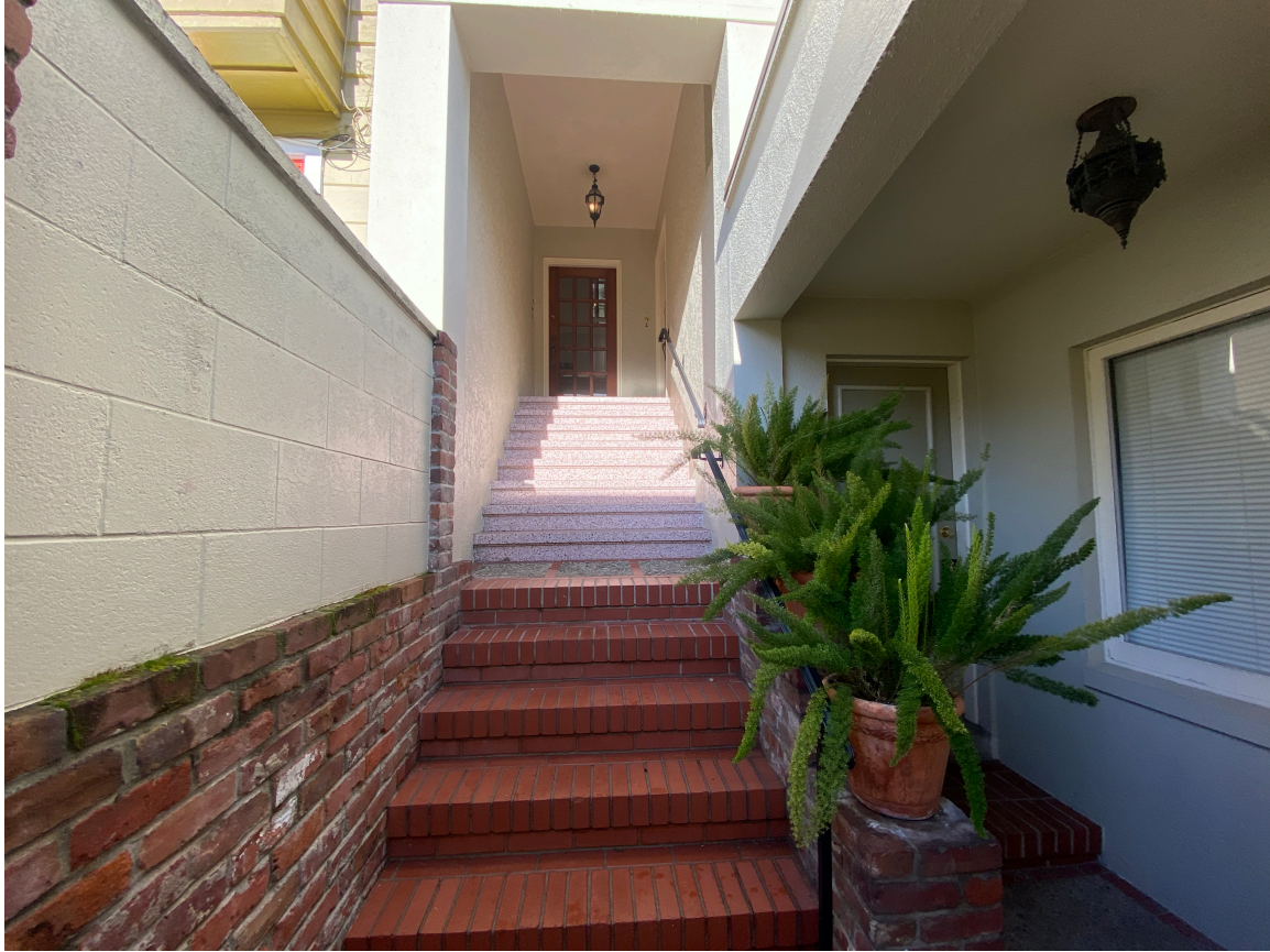
Fig 2: "Lightwell" to the right of the photo in question. One window with vision glass, and two solid doors (Second door to the right not shown in this view)
