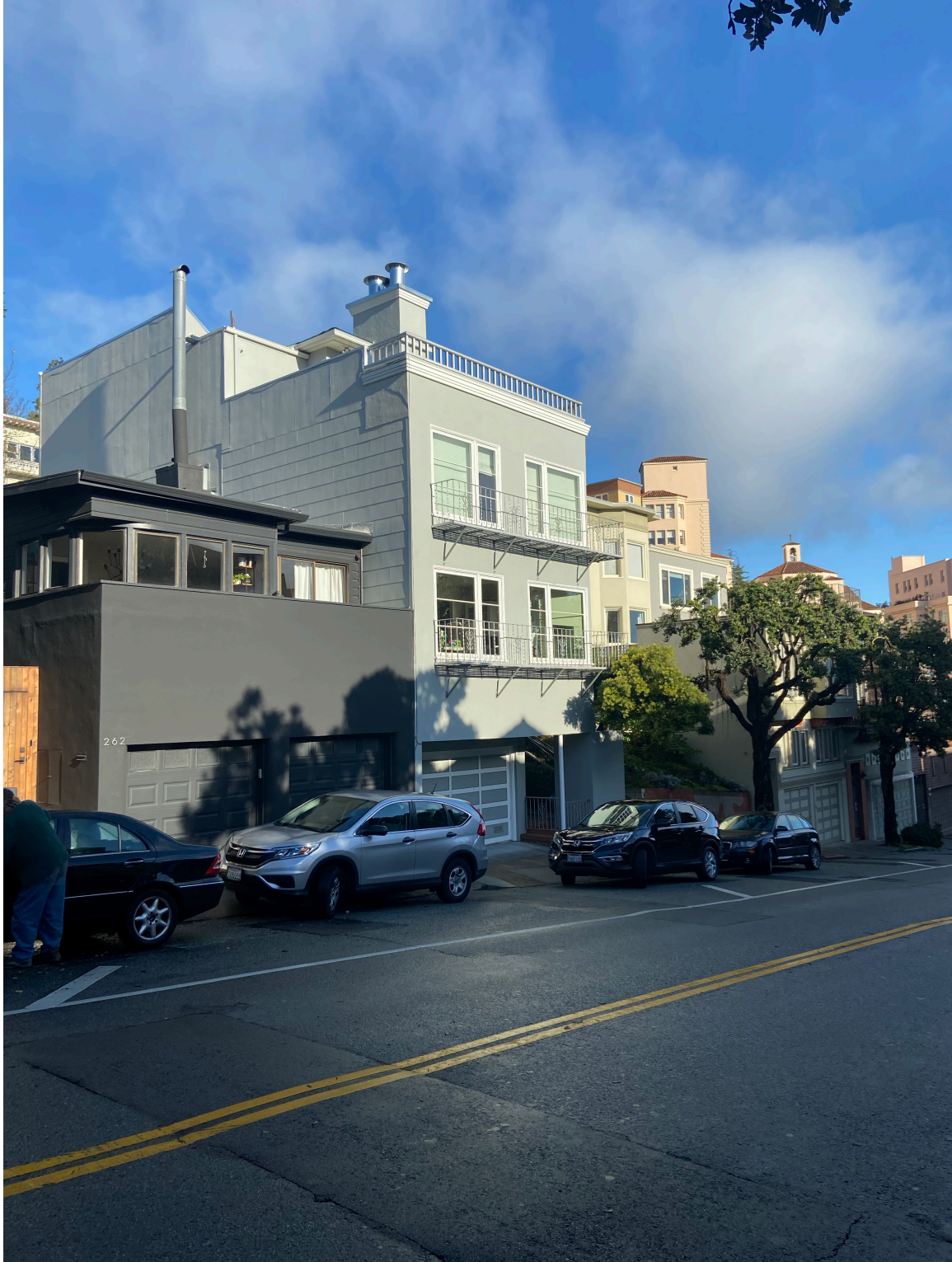
Fig 3: Transition between 262 and 258 Roosevelt does not step with topography
