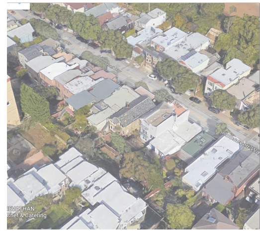
2. AERIAL PHOTO REAR OF PROPERTY LOOKING EAST
