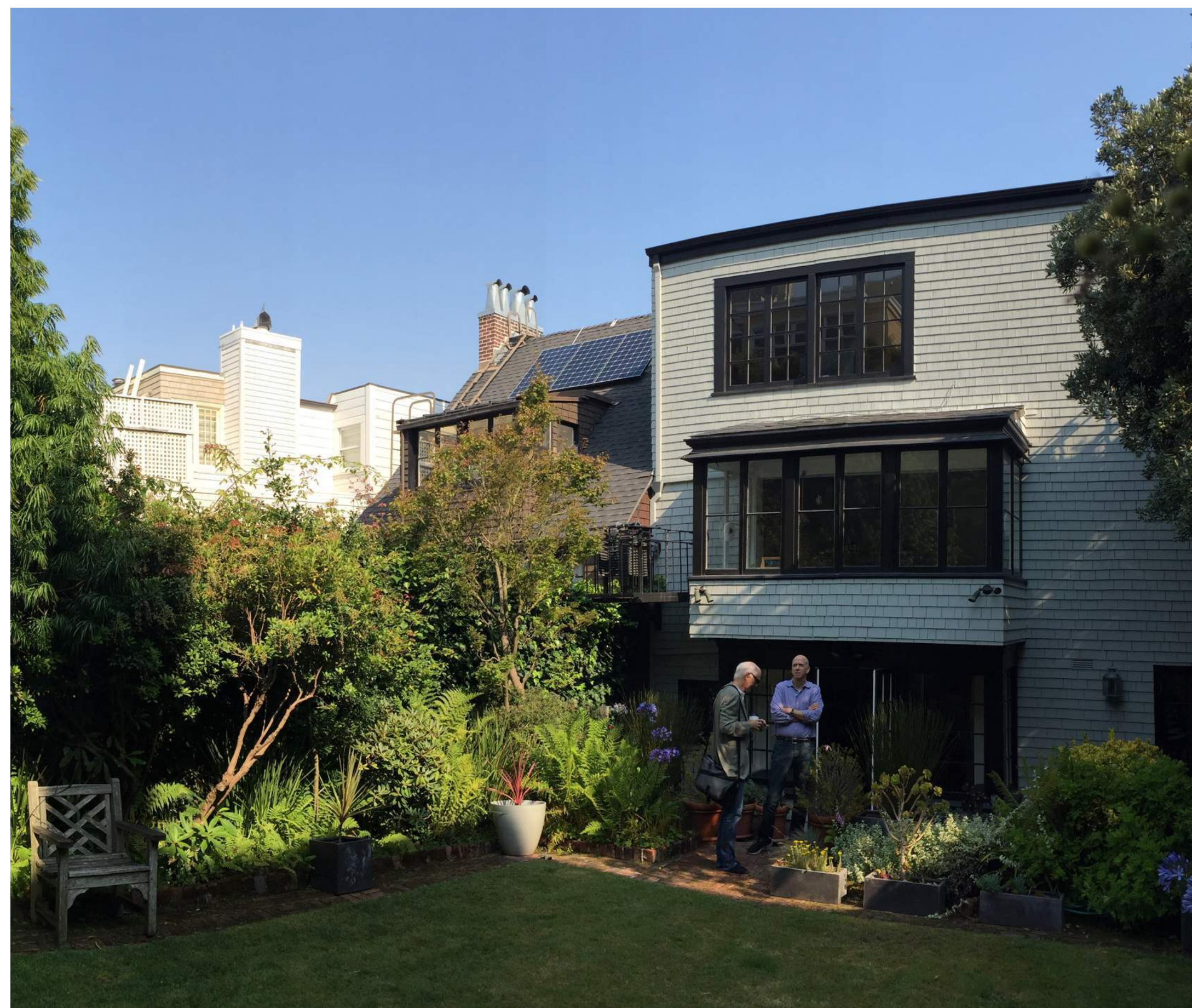
3 REAR YARD FACING NORTHWEST
