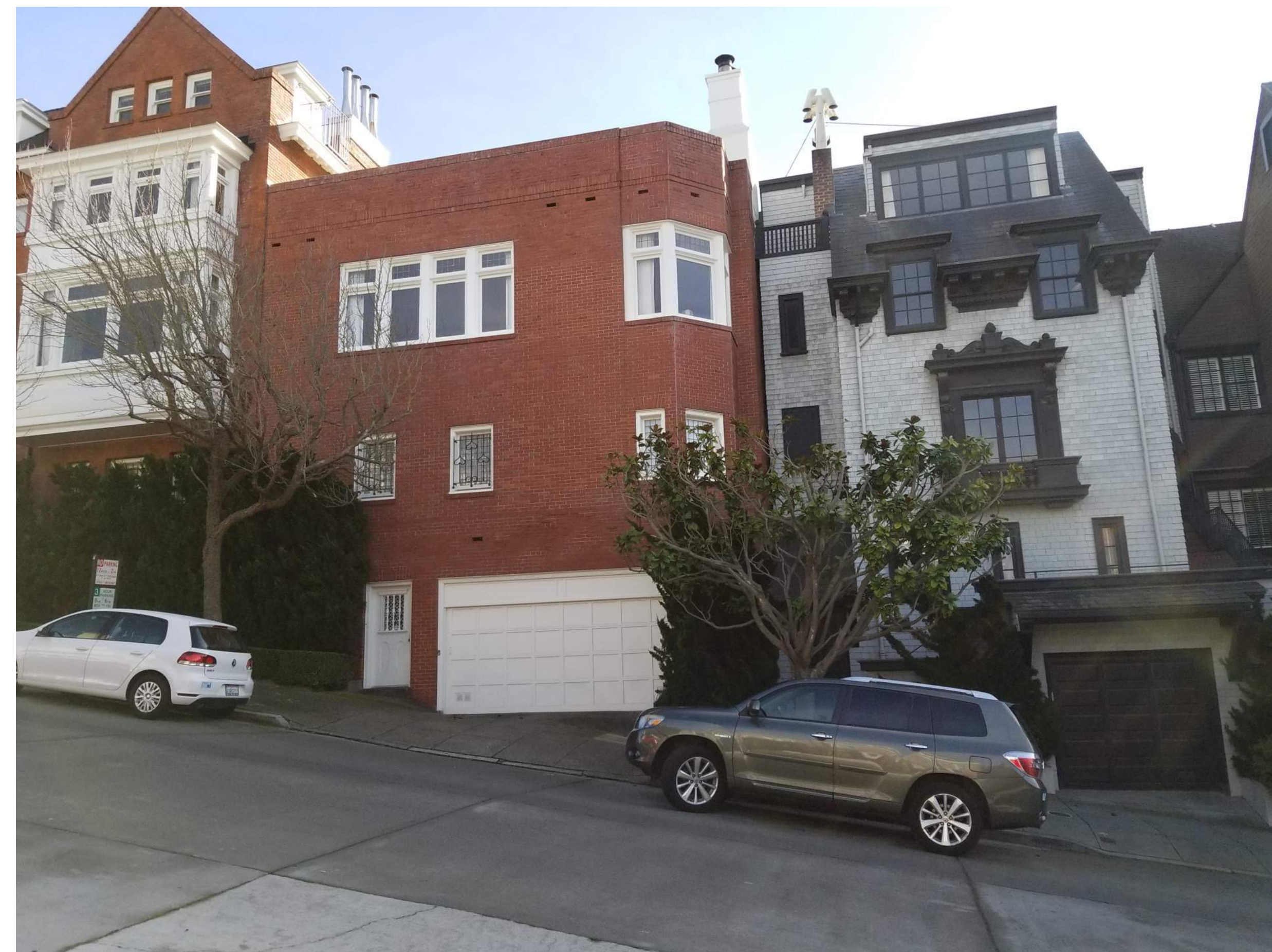
1 STREET FACADE FACING NORTH
