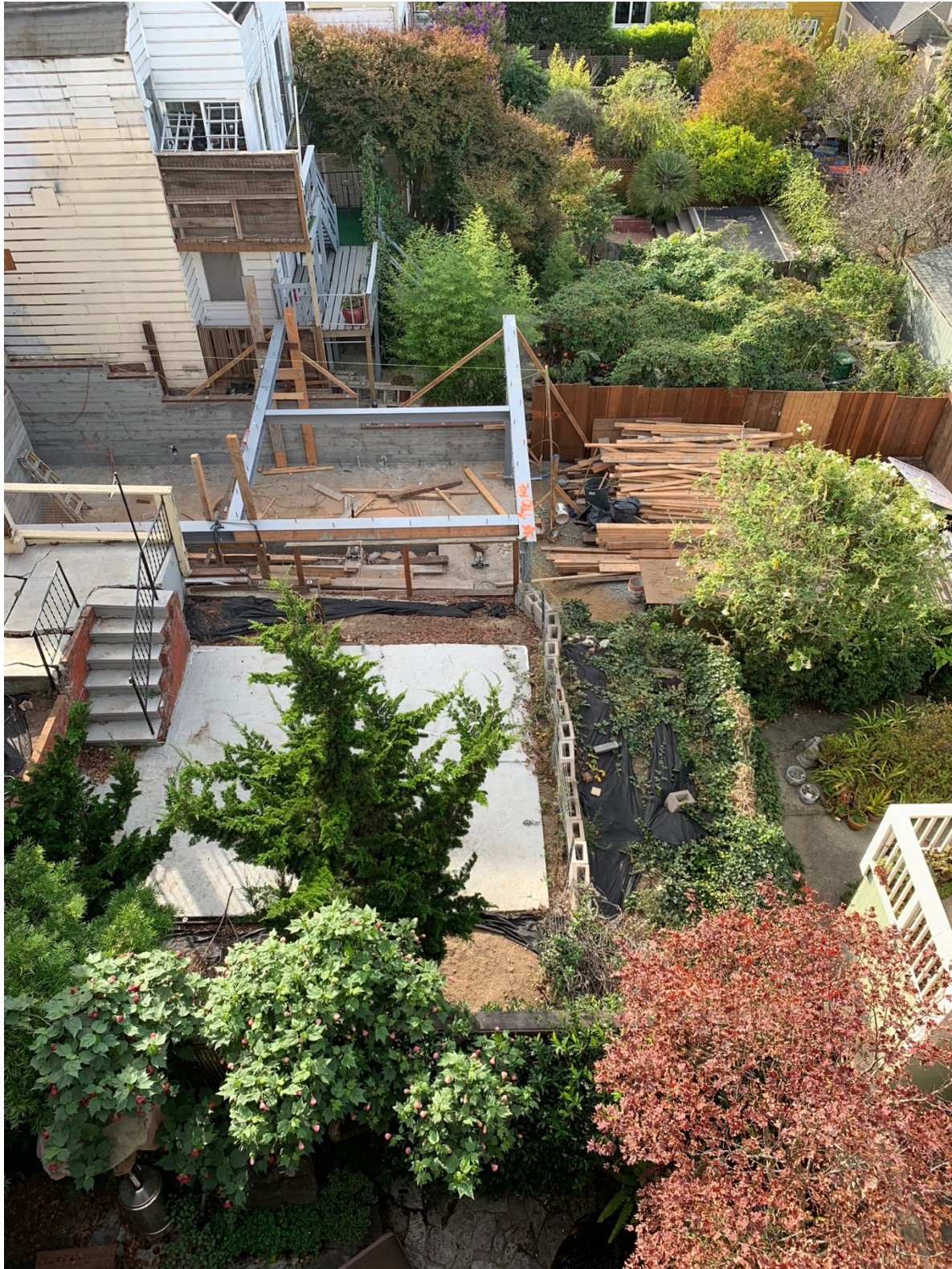
October 24, 2018 , under permit 2018-02272279 for interior remodel only. Note that new steel beam is outside the slab.
