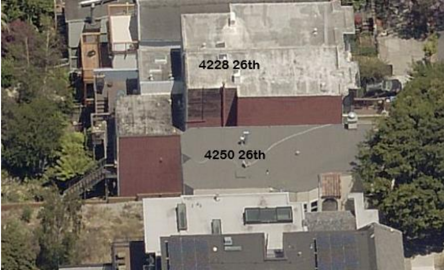
Figure 2. Aerial View from West
