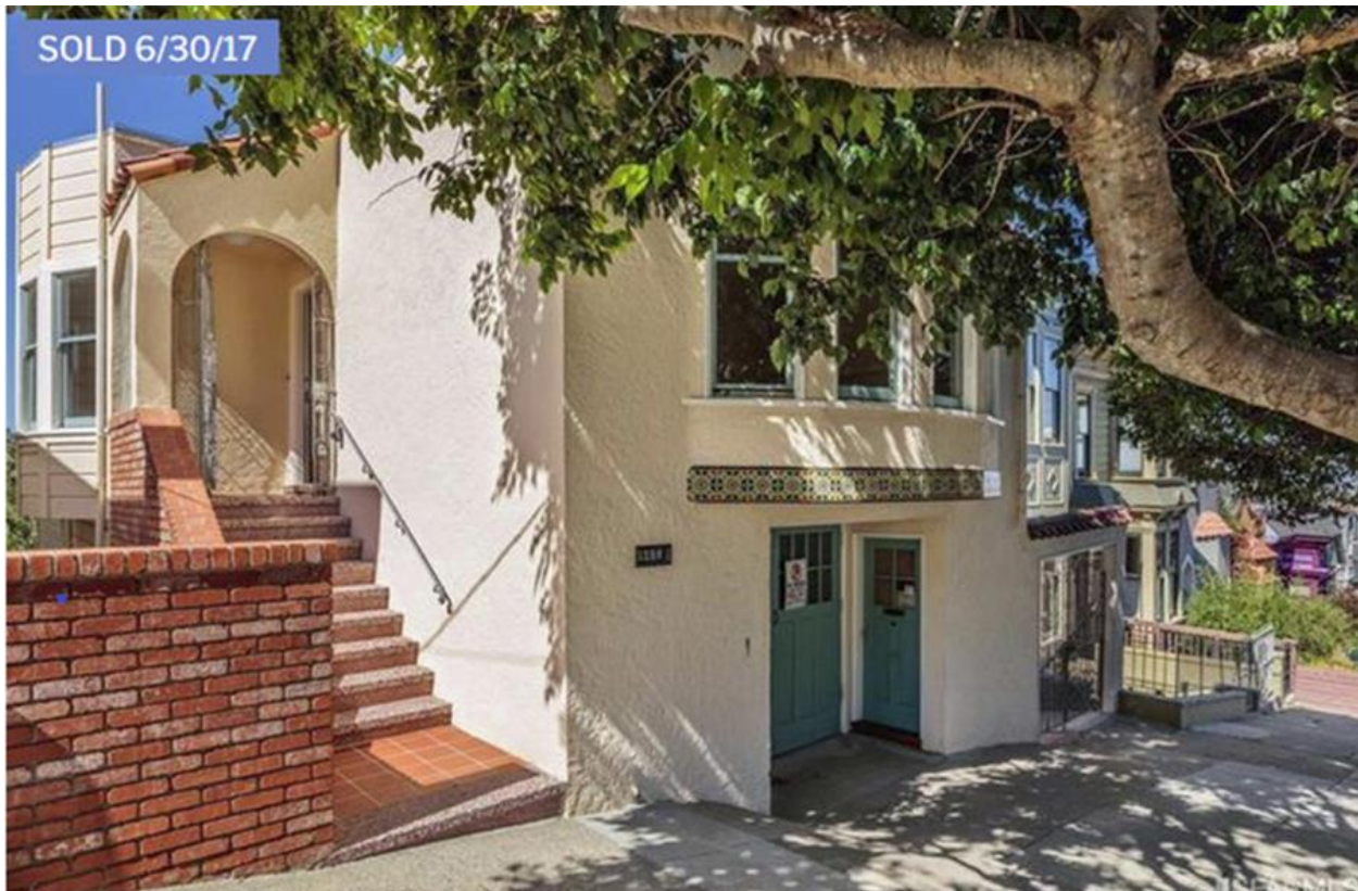
Figure 1. Existing Two-Story Home at 4250 26 th Street
