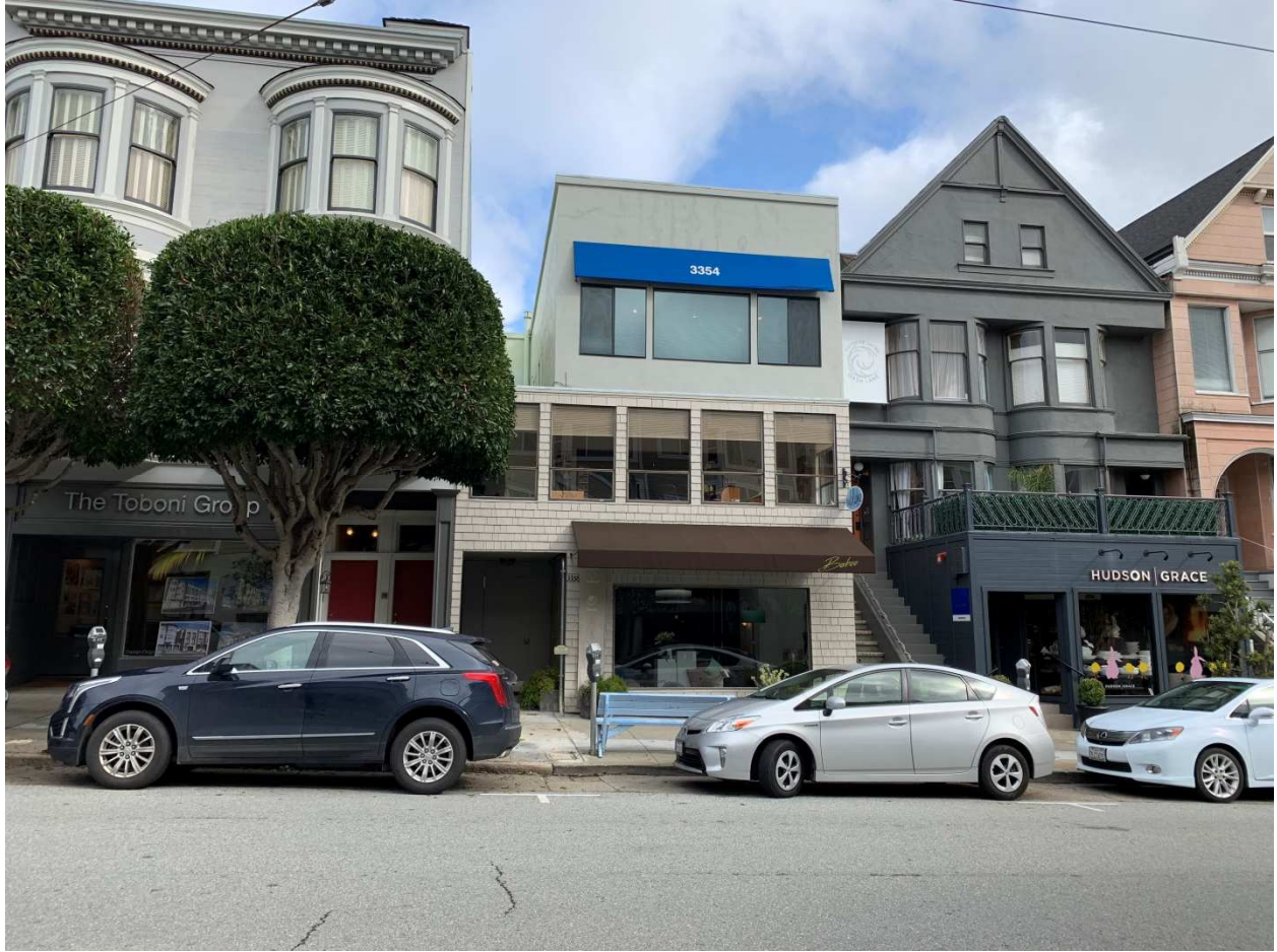
View of 3360 Sacramento from across the street
