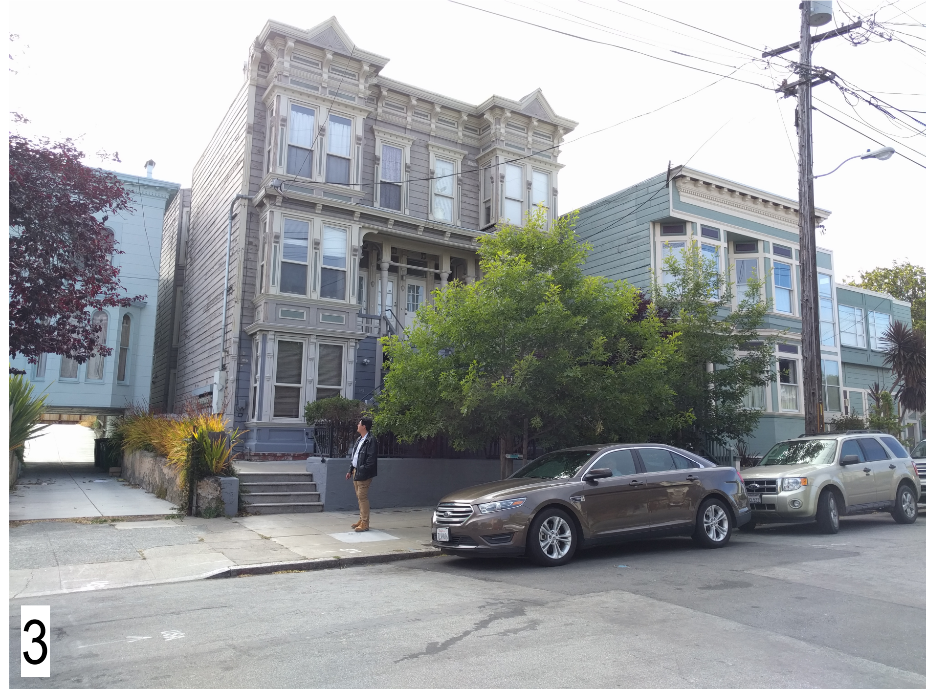
3-SUBJECT PROPERTY'S RIGHT VIEW
