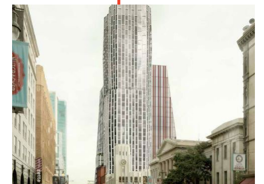
5M - FIVE NEW BUILDINGS
