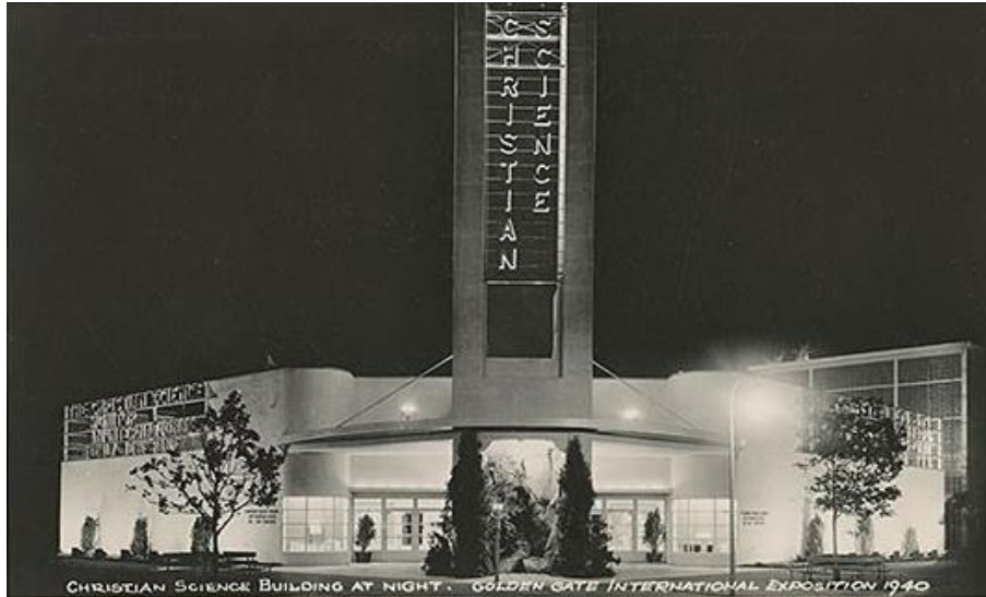
Figure 46: Christian Science Monitor Building, designed by Edward and John Bolles. Source: Treasure Island Museum GGIE postcard digital archive.
