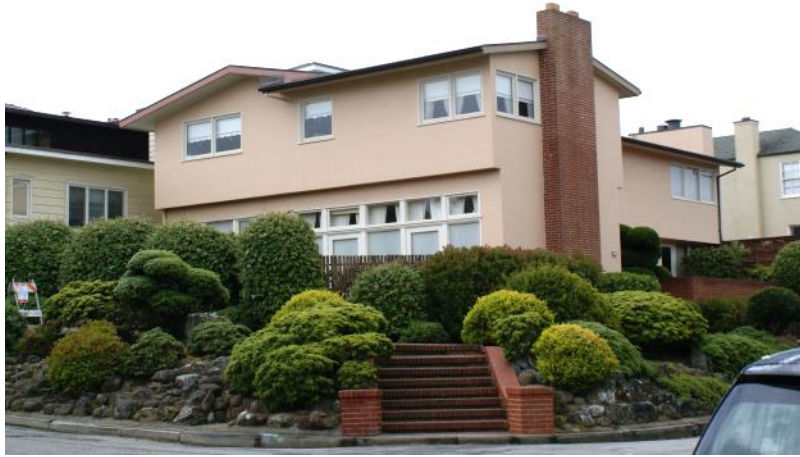
Figure 19: 201 Sea Cliff Avenue, southwest of the property across the street, constructed 1952.
