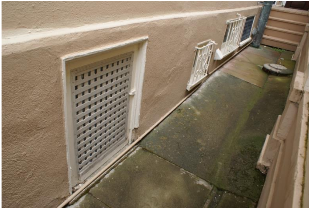
Figure 9: Partially exposed basement along the west façade, facing southeast.
