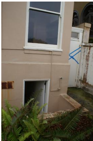
Figure 12: Subgrade basement entrance on the north façade, facing south.
