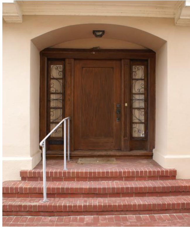
Figure 6: Primary entrance, facing west.
