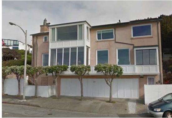
Figure 31: 475 Sea Cliff Avenue, constructed in 1971. Source: Google Maps Street view, 2017.
