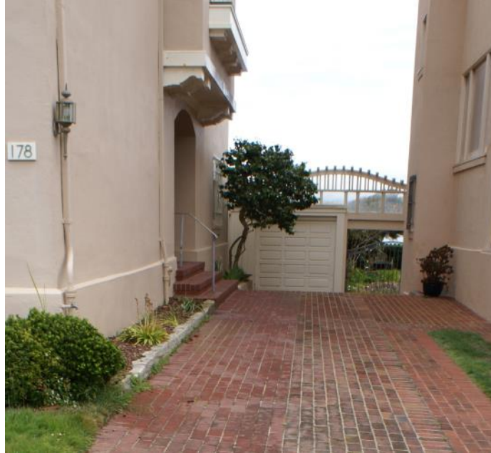
Figure 13: Front entrance of the garage, facing north.
