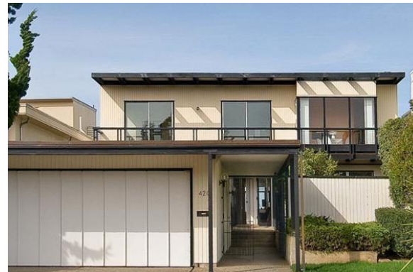
29. 420 EL CAMINO DEL MAR (1958/2014) BY JOE ESHERICK (1958) REMODELED BY EDMONDS+LEE ARCHITECTS (2014)
