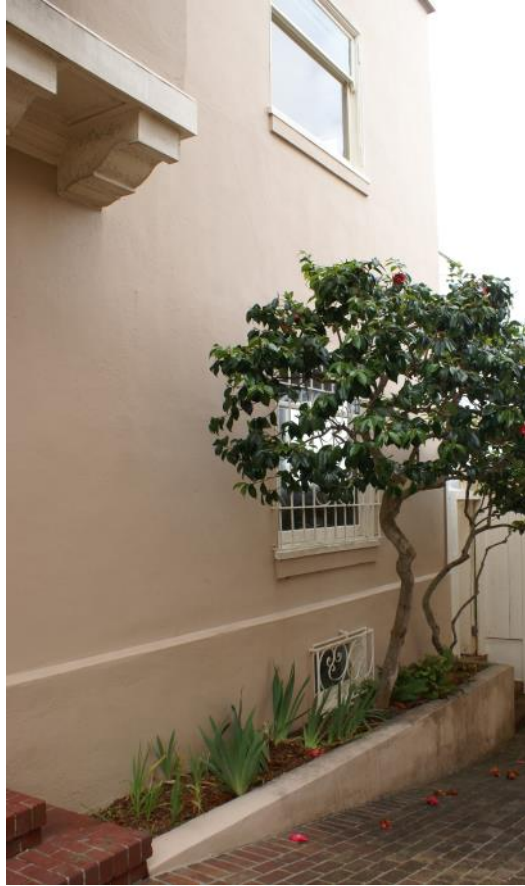
Figure 7: Lower right of east façade, facing northwest.
