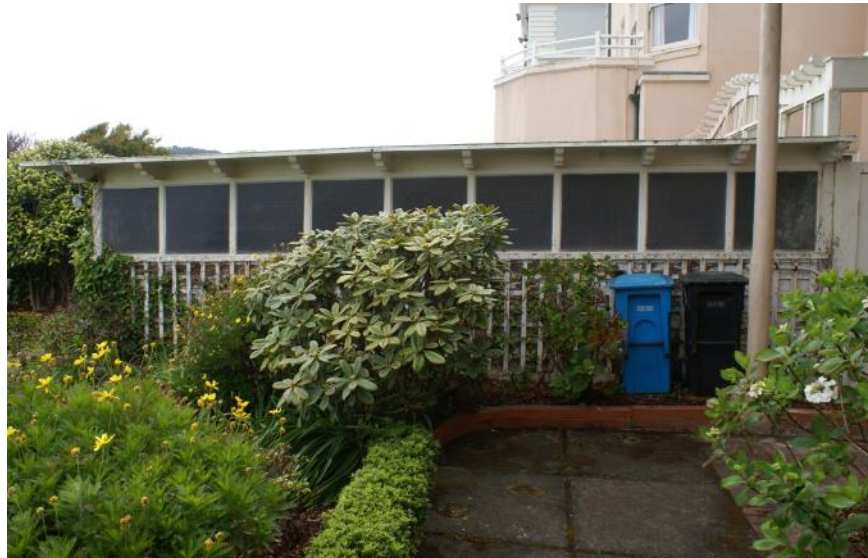
Figure 14: West façade of the garage, facing east.
