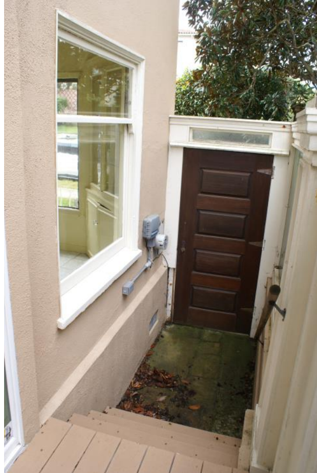
Figure 10: Southern portion of the west façade, facing south.
