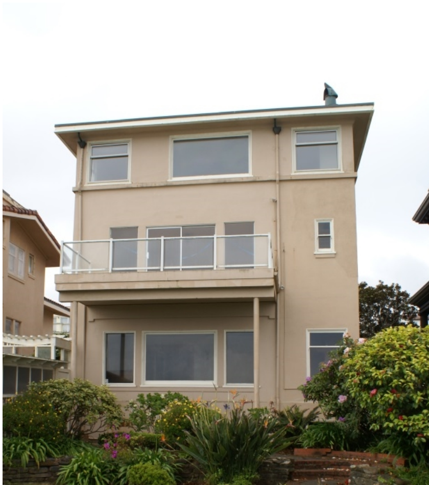
Figure 11: North façade and garden, facing south.
