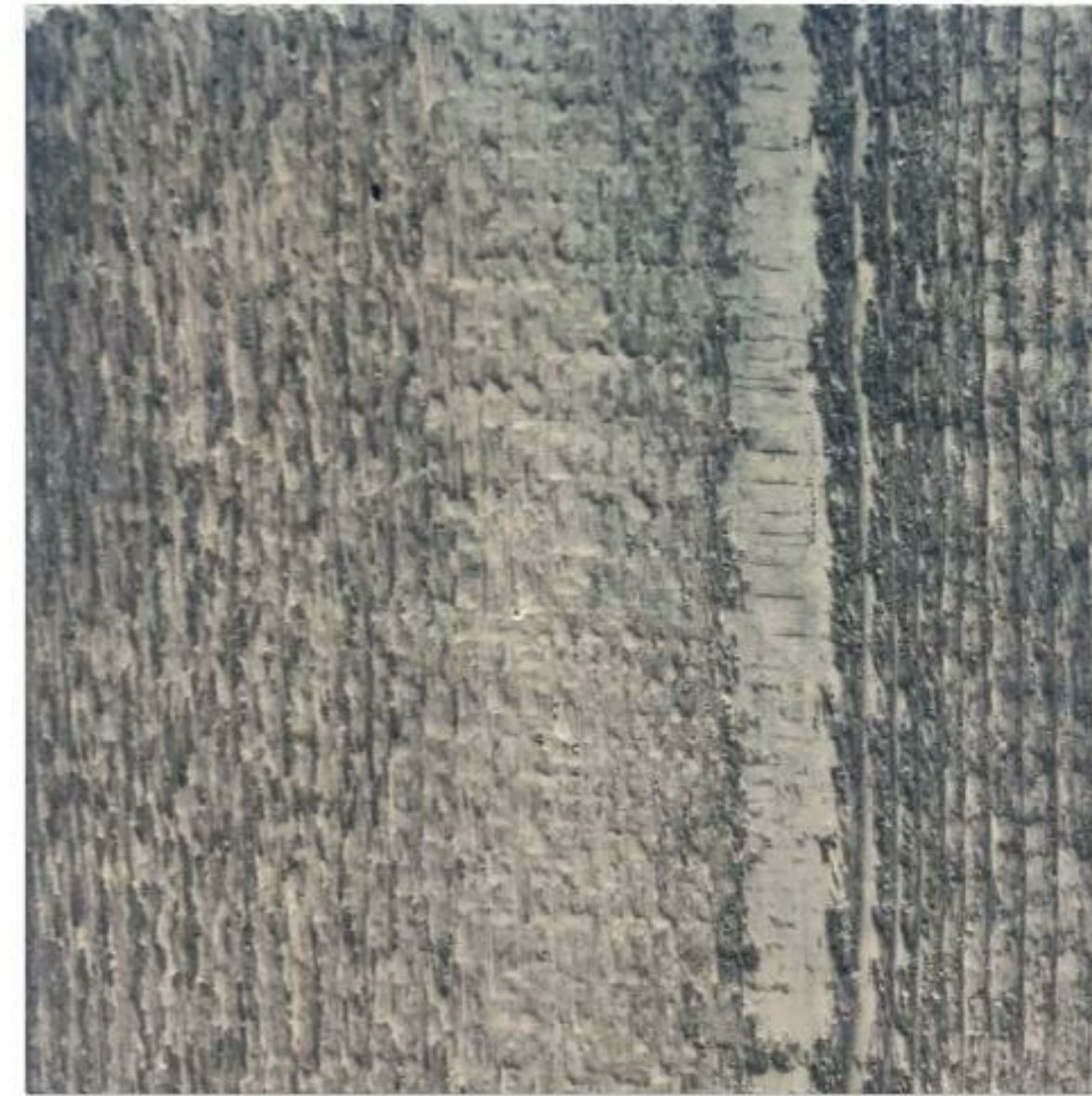
BOARD FORM CONCRETE (SAMPLE FOR TEXTURE ONLY) ③
