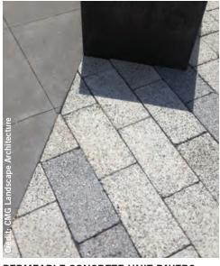
PERMEABLE CONCRETE UNIT PAVERS
