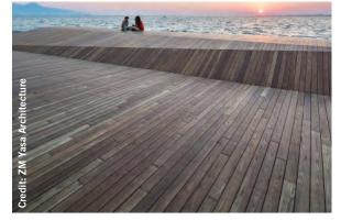
Wood decking made of durable hardwood appropriate for coastal conditions.
