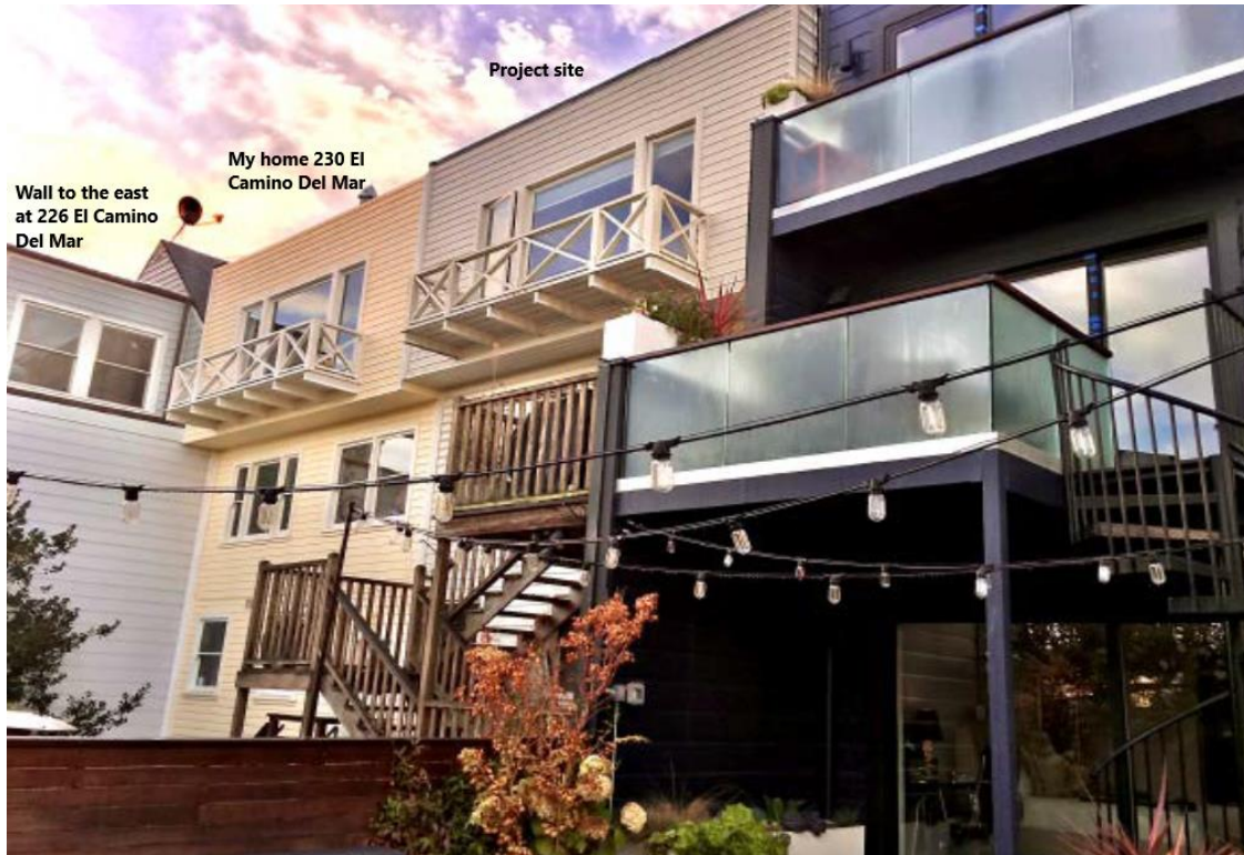
Figure 5. Existing 15-foot deep wall adjacent and to the east of my home – View 1
