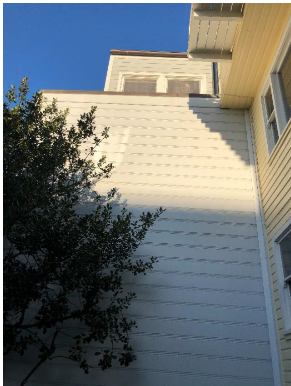
Figure 6. Existing 15-foot deep wall adjacent and to the east of my home – View 2
