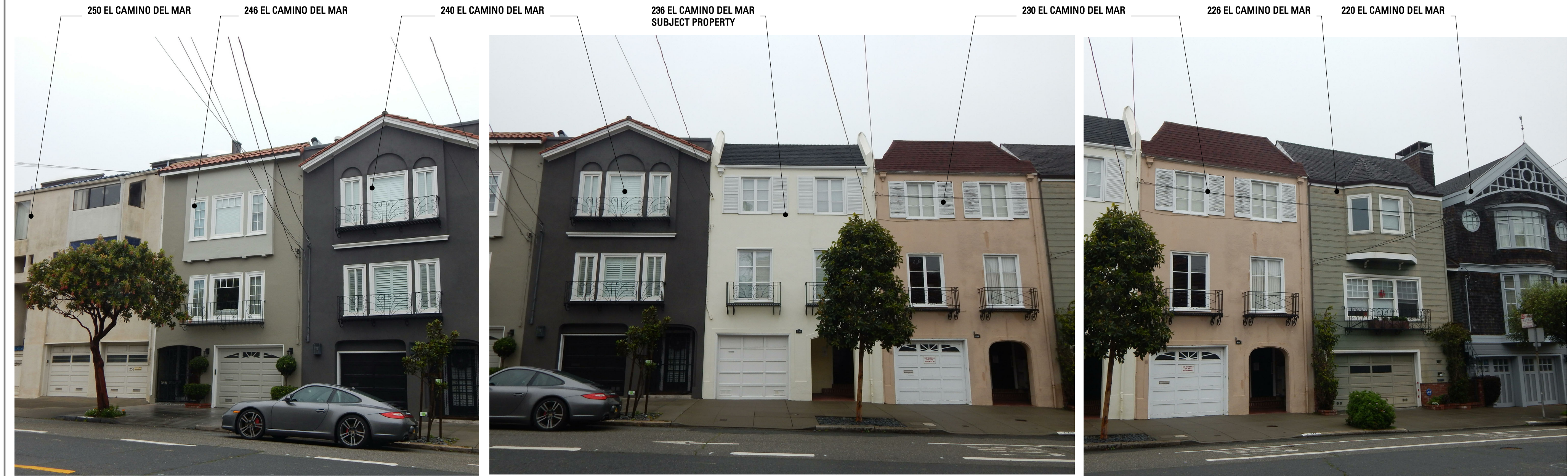
(E) SITE PHOTOS - FRONT YARD VIEW
