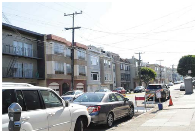
1 EXISTING BUILDING (OBLIQUE ANGLE VIEW FORM NORTH)
