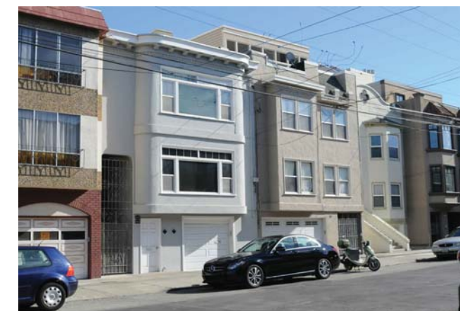
4 PROPOSED BUILDING (CLOSE UP VIEW FORM NORTH)
