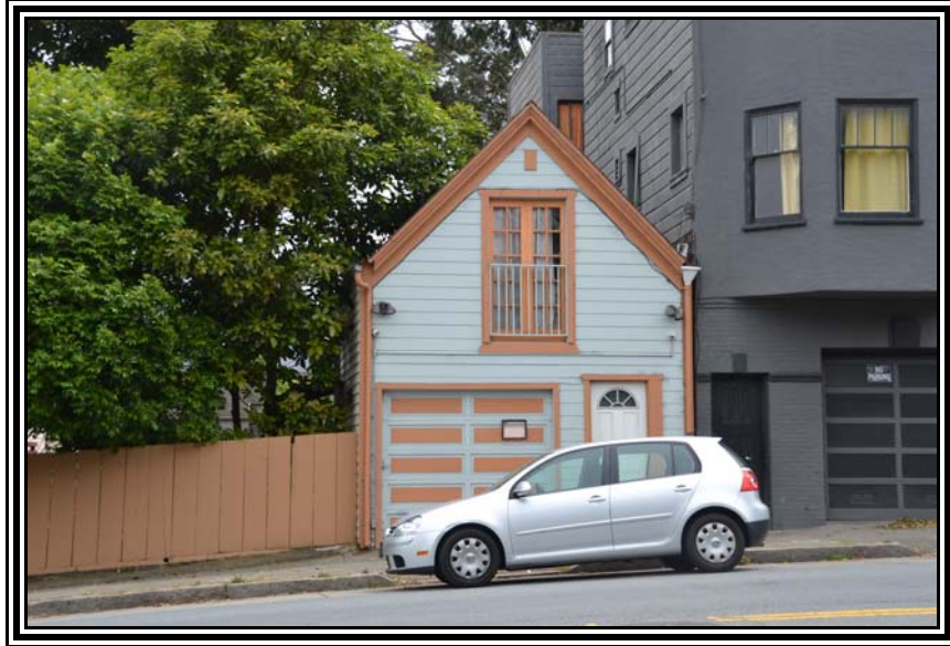
Building at rear (west end) of lot. While the garage door is there, there is no garage inside.
