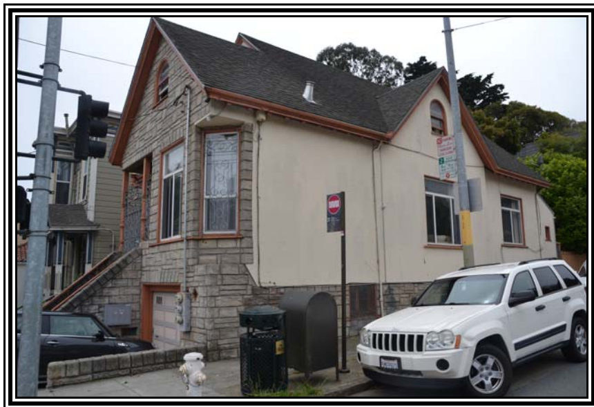
Subject Property from Turk Street
