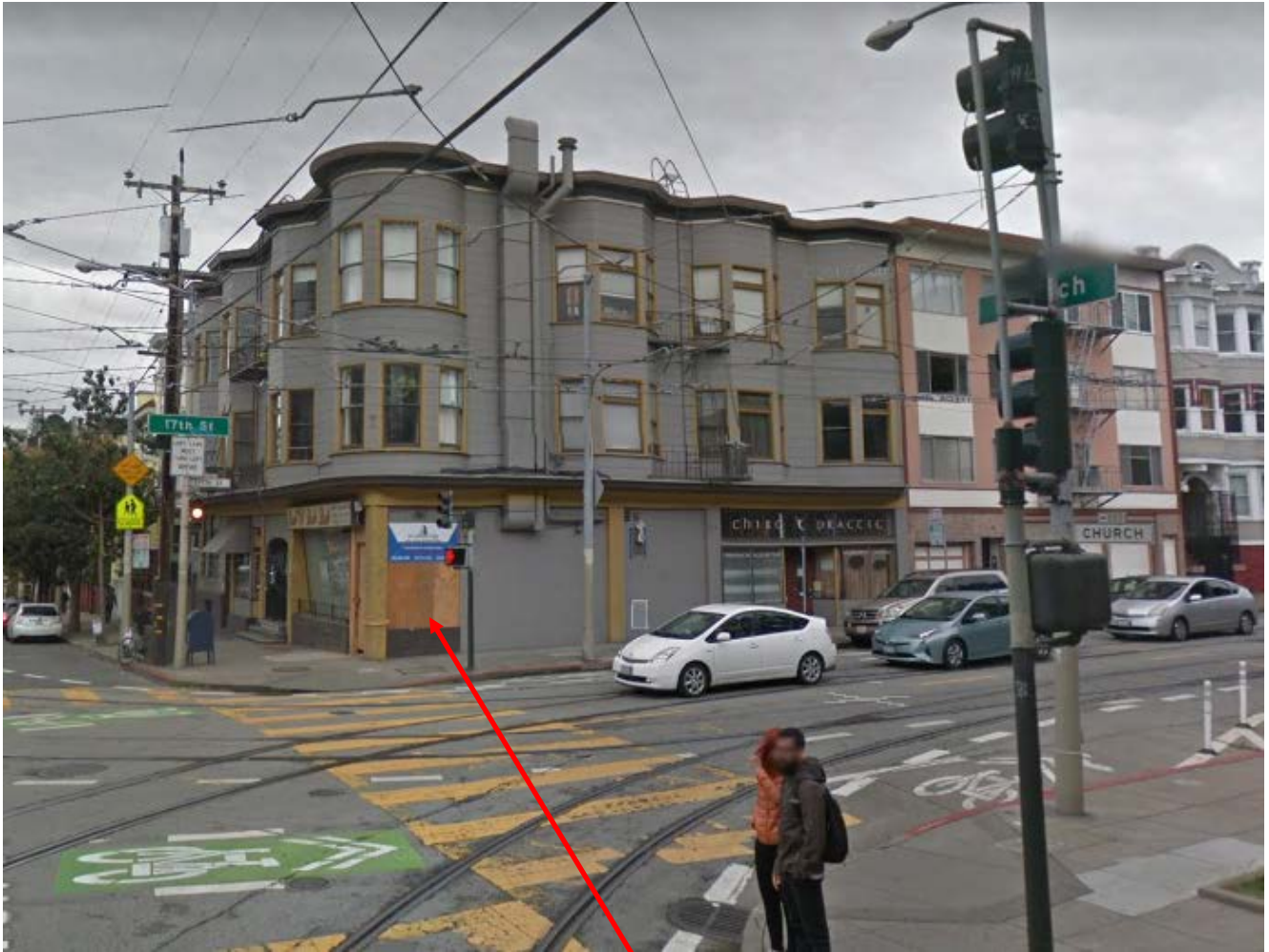
SUBJECT PROPERTY - VIEW LOOKING NORTH ON CHURCH STREET
