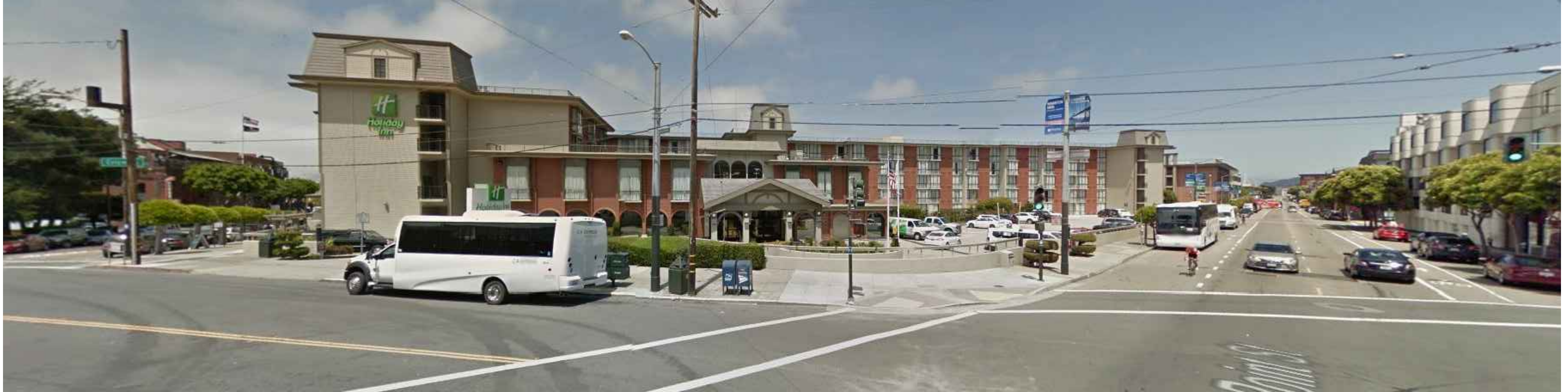
VIEW LOOKING NORTHEAST ALONG NORTH POINT ST.
