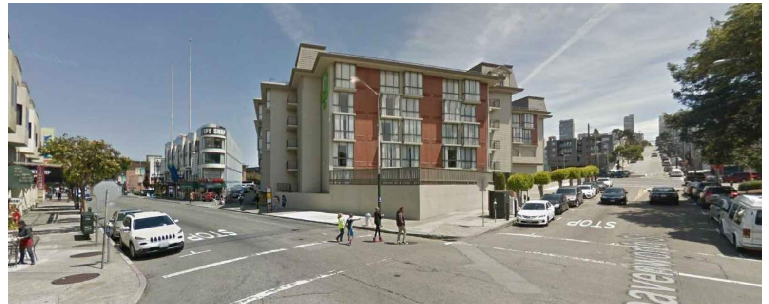
VIEW LOOKING SOUTHEAST ALONG LEAVENWORTH ST.
