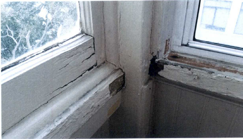
Mold and Dry Rot in Unit 6 Sunroom
