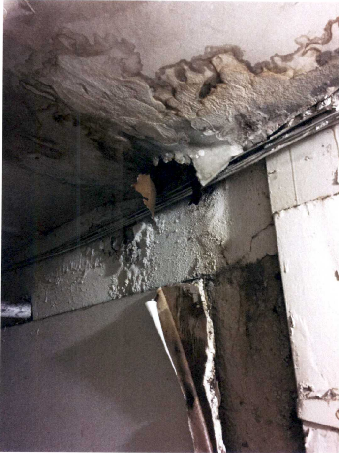
Corroded and Moldy / Fungal Ceiling Above Storage Unit
