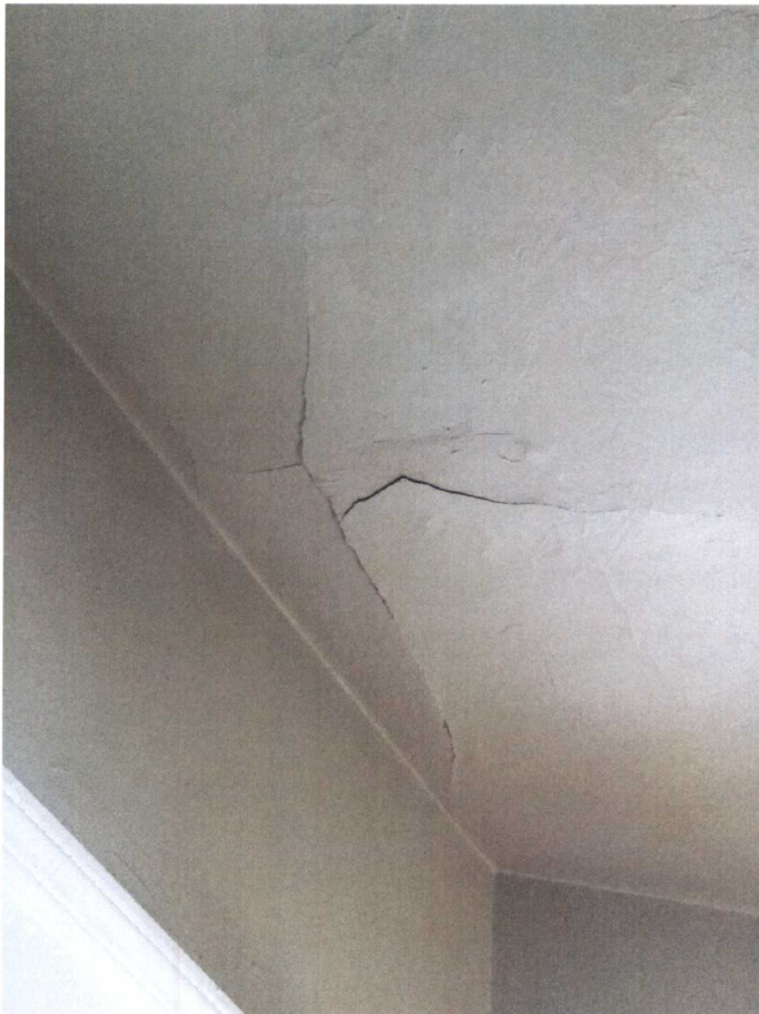
Ceiling Damage From Leaks, Unit 9
