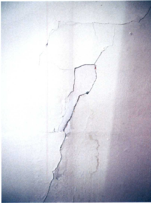
Similar Radiator Steam Damage, Unit 10
