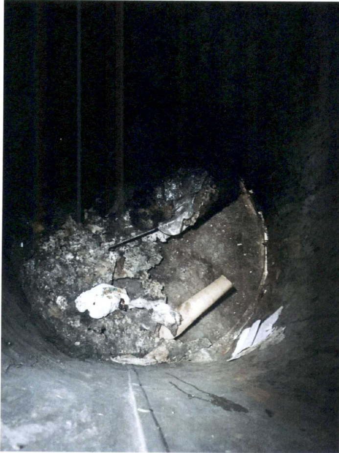
Broken and Corroded Bottom of East Side Common Garbage Bin
