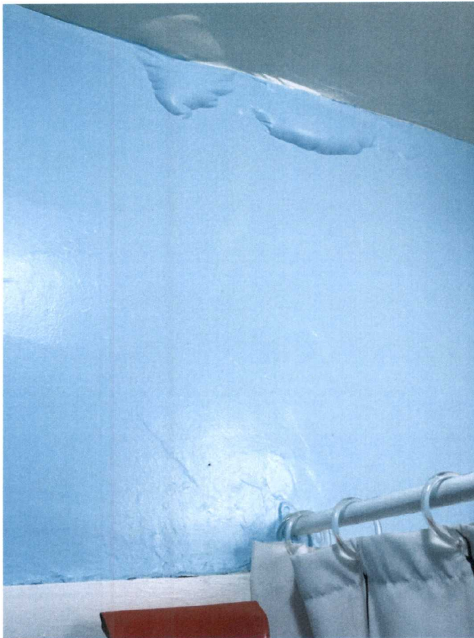
Leak Blisters, Bathroom Wall, Unit 4
