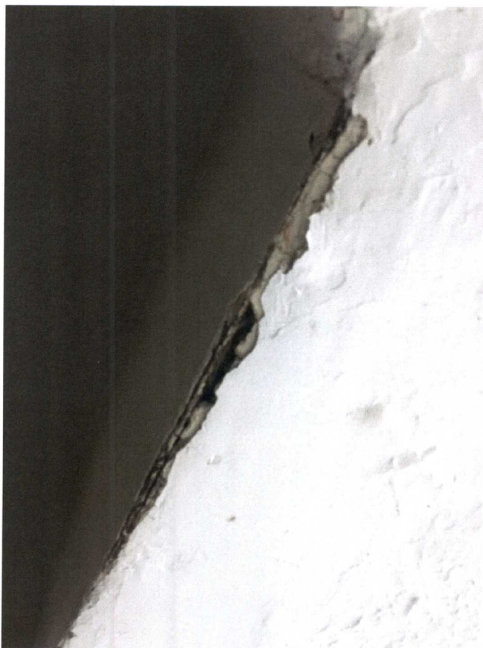
Ceiling Peeling Away Above Foot of Stairs
