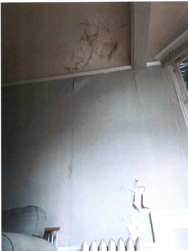
Radiator Steam Damage Unit 4
