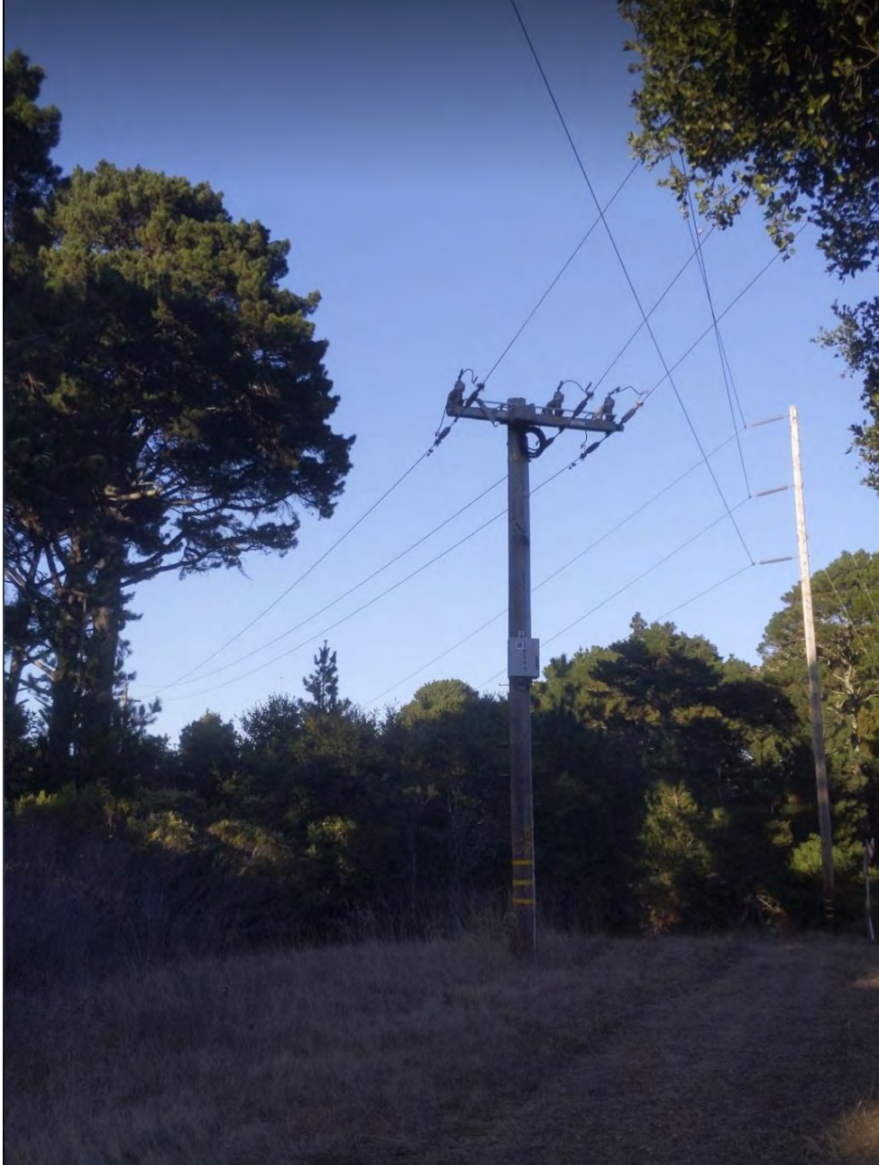
Photo taken in SF Watershed near HWY 92 and Old Canada Road
